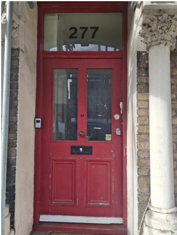
Ground Floor Rear Exit Door
