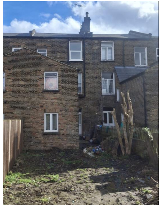
No 279 Rear Elevation (West)
