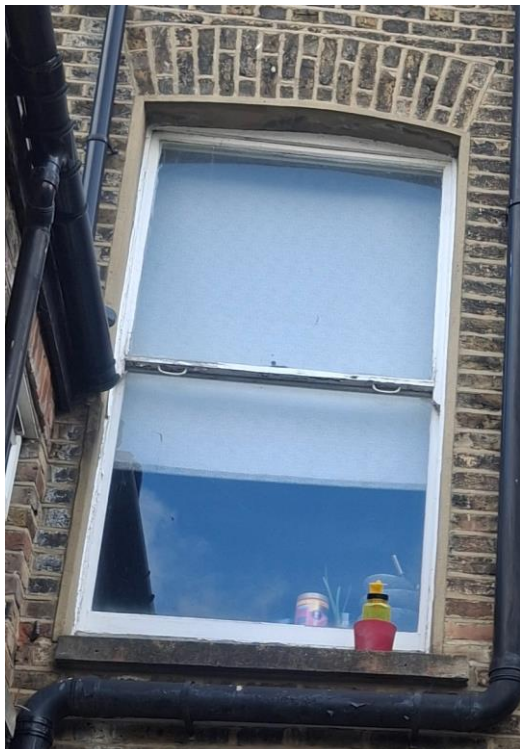
Rear First Floor Window (279)
