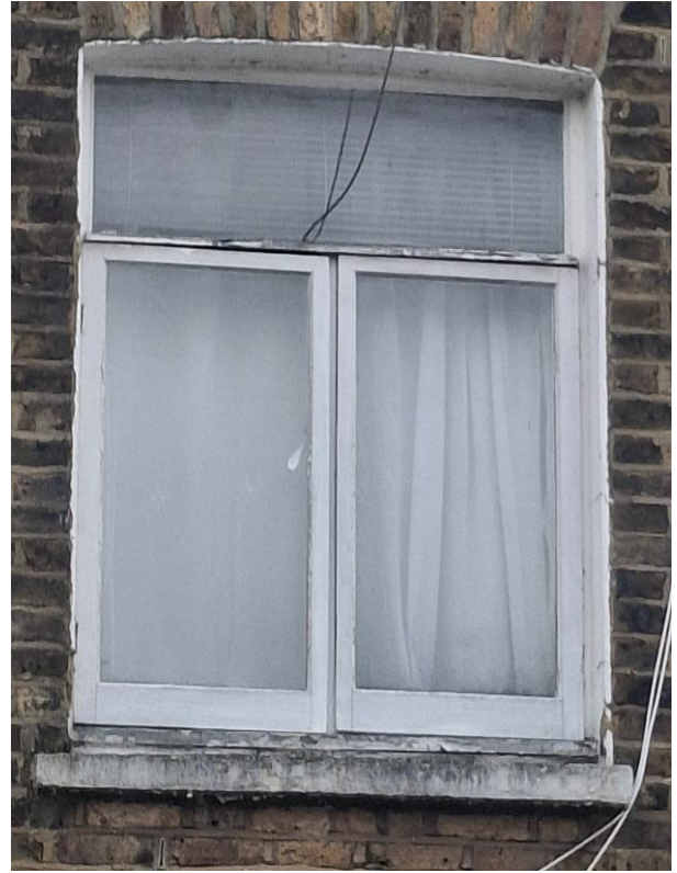
Rear End First Floor Window (277)
