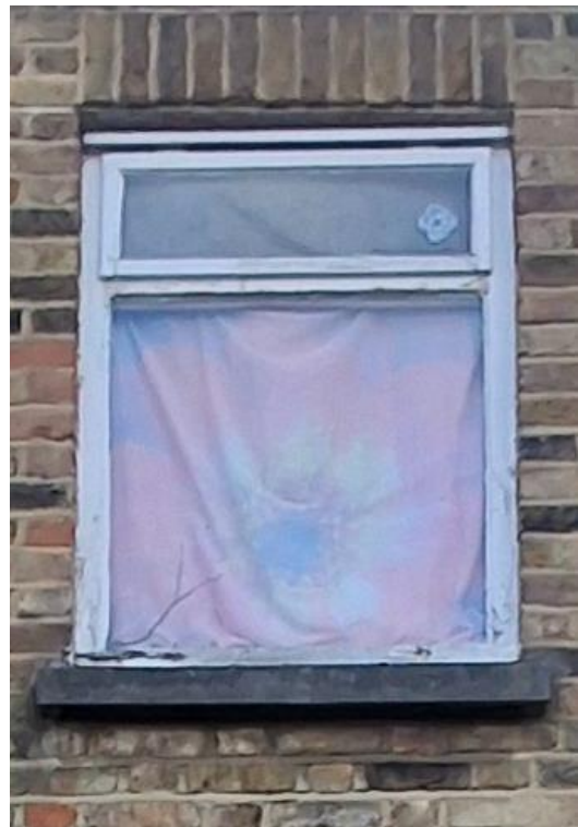
Rear End First Floor Window (279)
