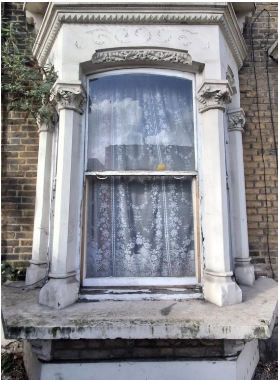
Front Ground Floor Bay Window (279)
