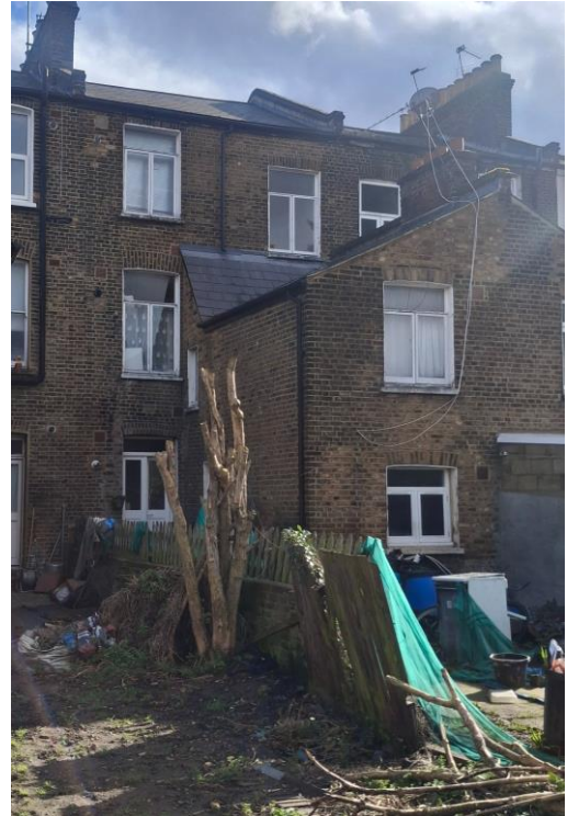
No 277 Rear Elevation (West)
