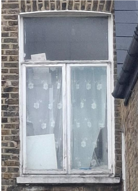
Rear First Floor Window (277)
