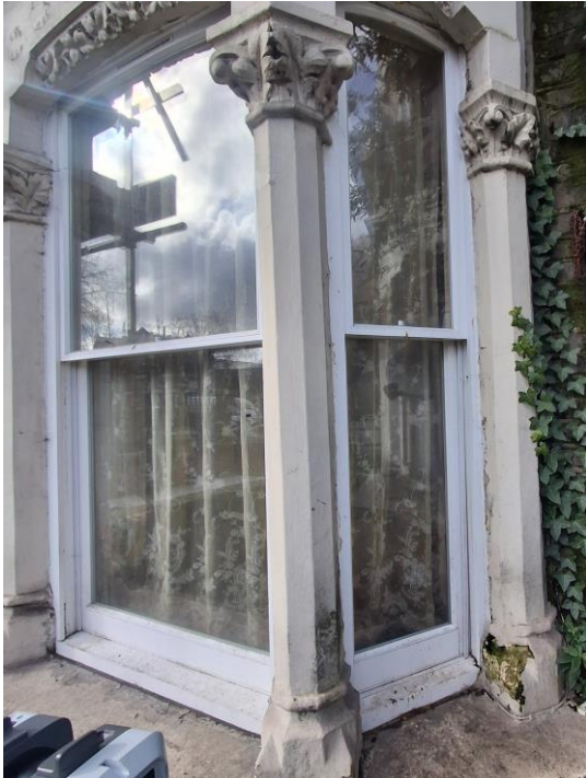
Front Ground Floor Bay Window (277)
