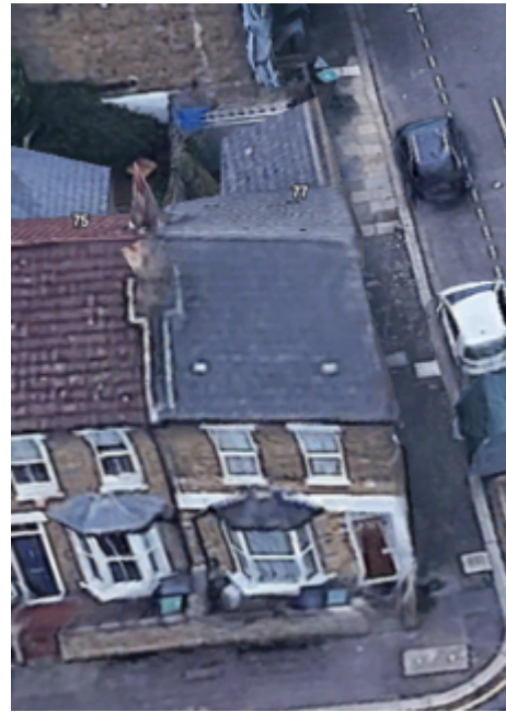
Roof Front Elevation (North)
