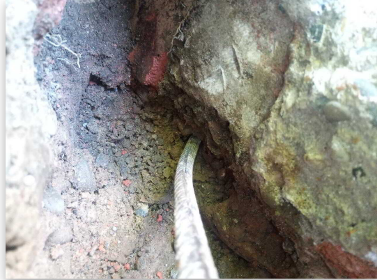
Fig 1.2: Trial Hole 1 Footing
