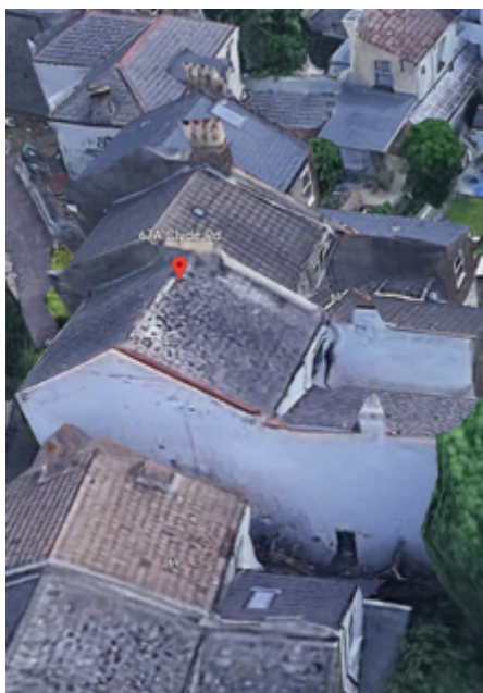
Roof Side Elevation (West)
