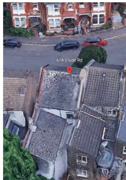
Roof Rear Elevation (South)
