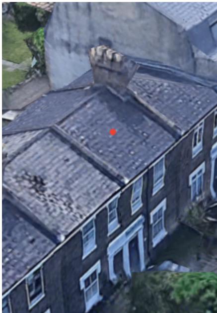
Roof Side Elevation (North)
