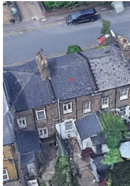
Roof Rear Elevation (East)
