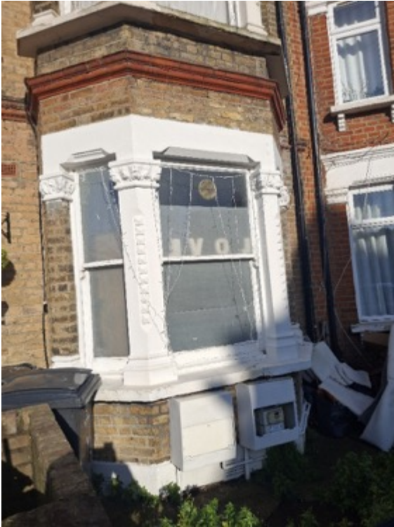
Windows (ground floor – front elevation)
