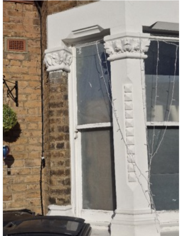
Windows (ground floor – front elevation)
