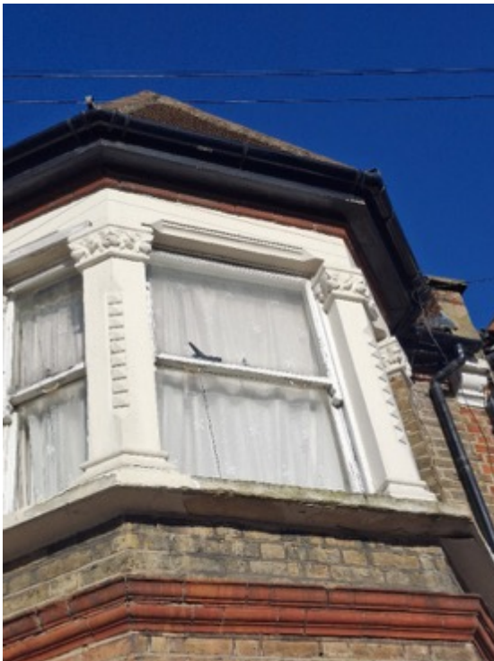
Window (Upper floors – front elevation)
