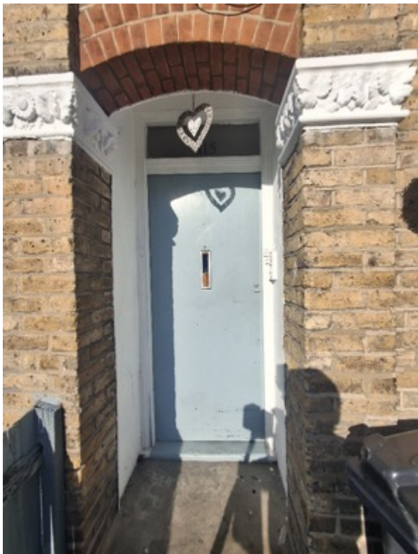
Existing Entrance Door
