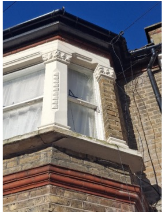
Window (Upper floors – front elevation)
