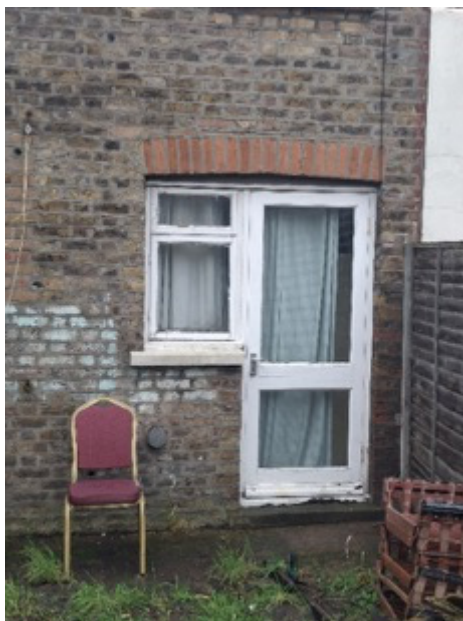
Back Exit Door 1
