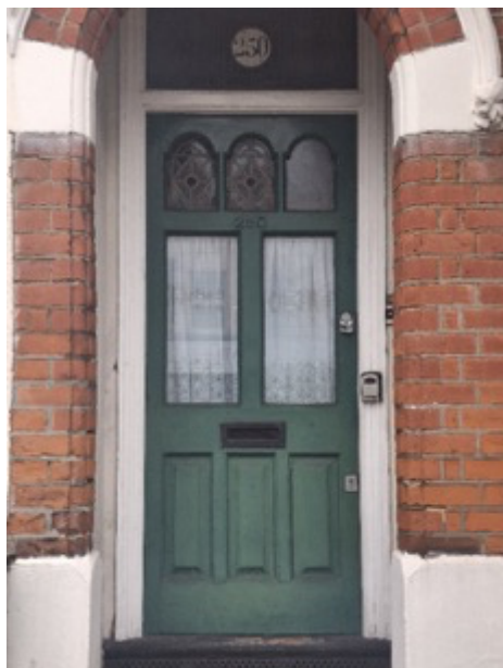
Front Entrance Door
