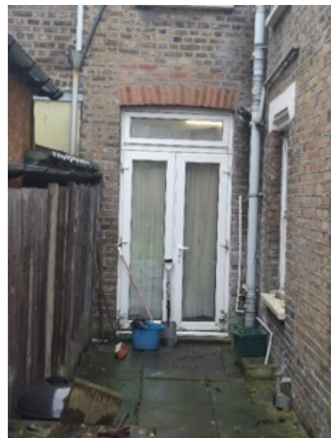
Back Exit Door 2
