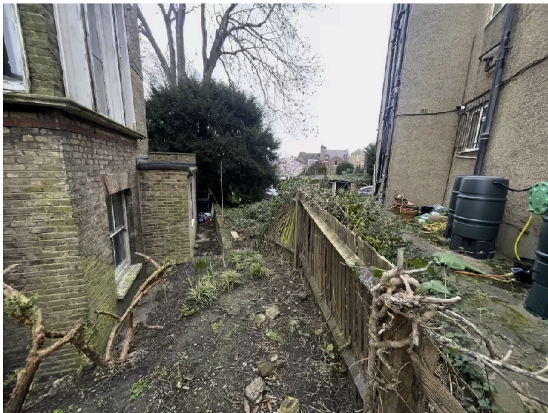
Illustrating the already close proximity between Elm Court and the bedroom windows of 53 Cholmeley Park at ground floor level and raised ground floor level. This also illustrates the parallel vertical walls which create vertical amplification of sound.
