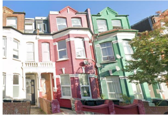
2) Front View of the Site at 59 Hampden Rd
