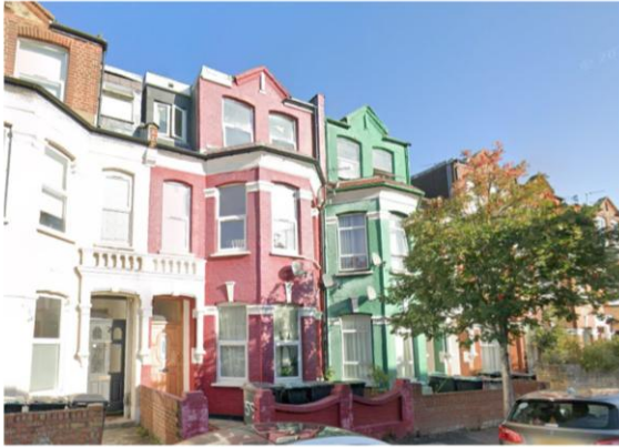
1) Front View of the Site at 59 Hampden Rd
