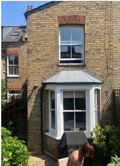
view of rear elevation
