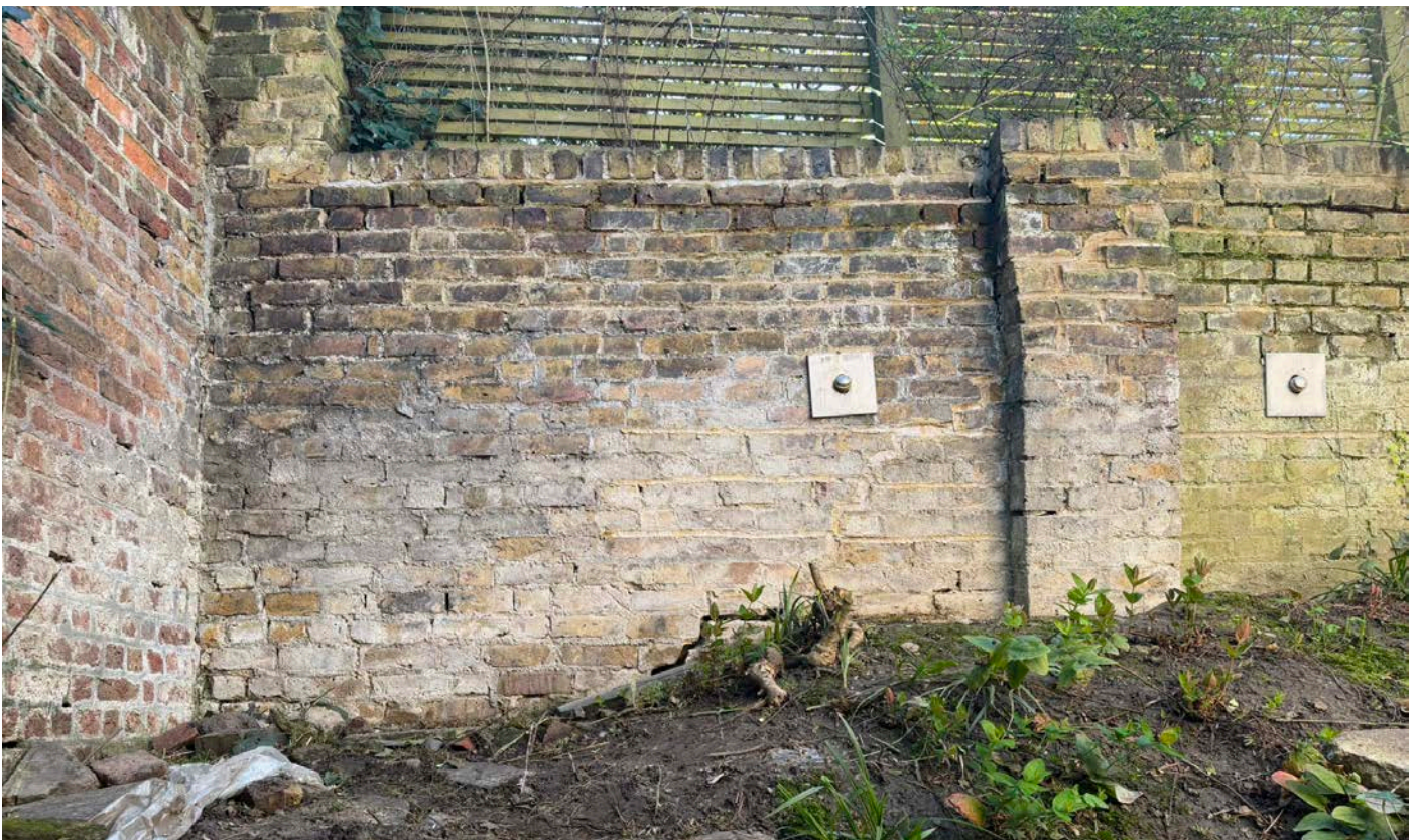
Photograph C - Cleaned section of existing boundary wall in a dry state.
