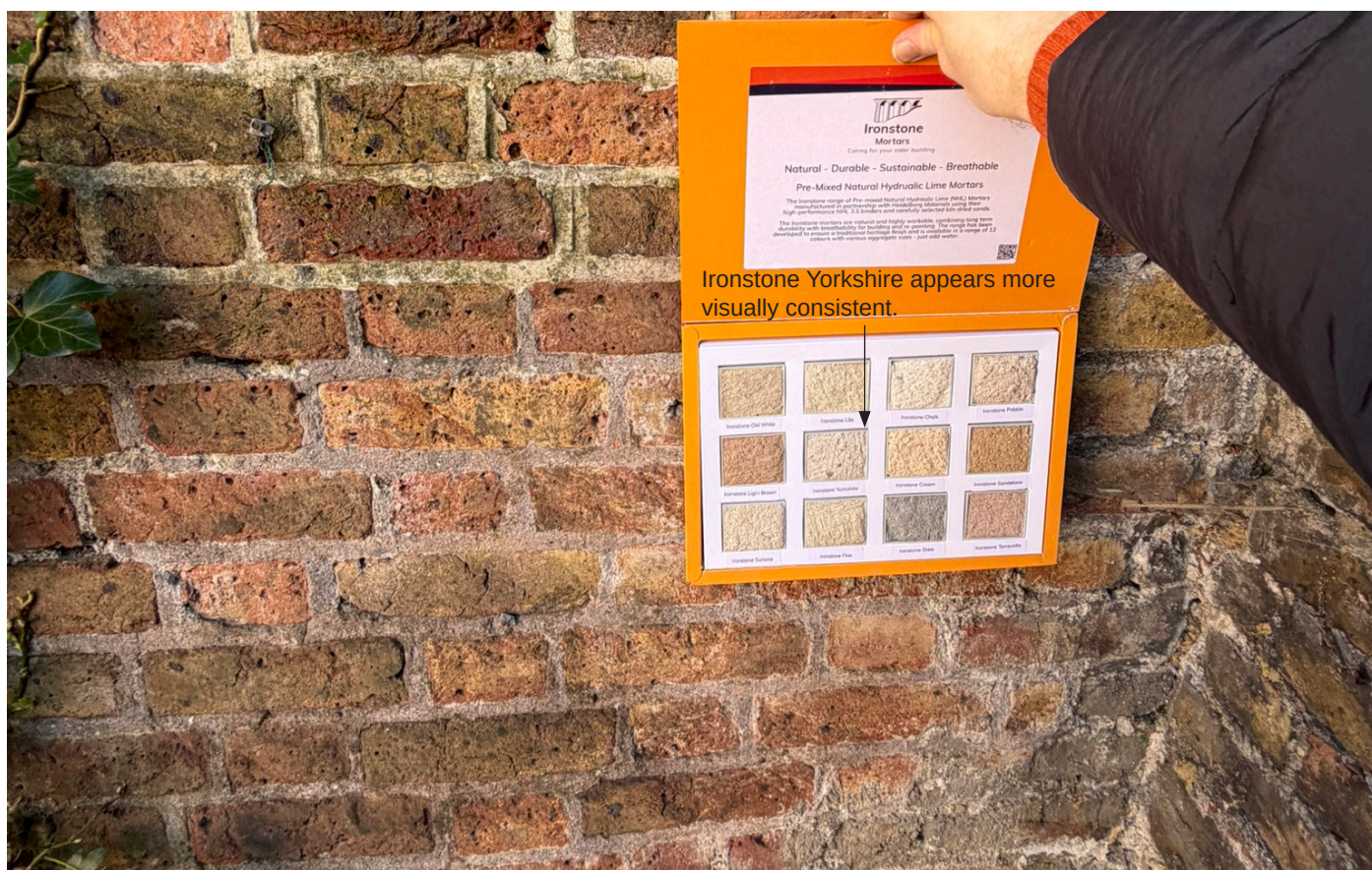
Photograph N Comparison of mortar in underpinned wall perpendicular to the South boundary wall to be rebuilt.
