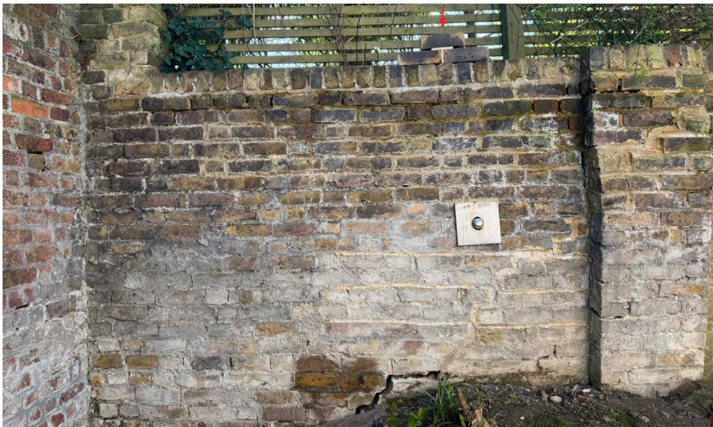
Photograph H - Photograph of tinted Danehill Yellows at the top of the boundary wall
