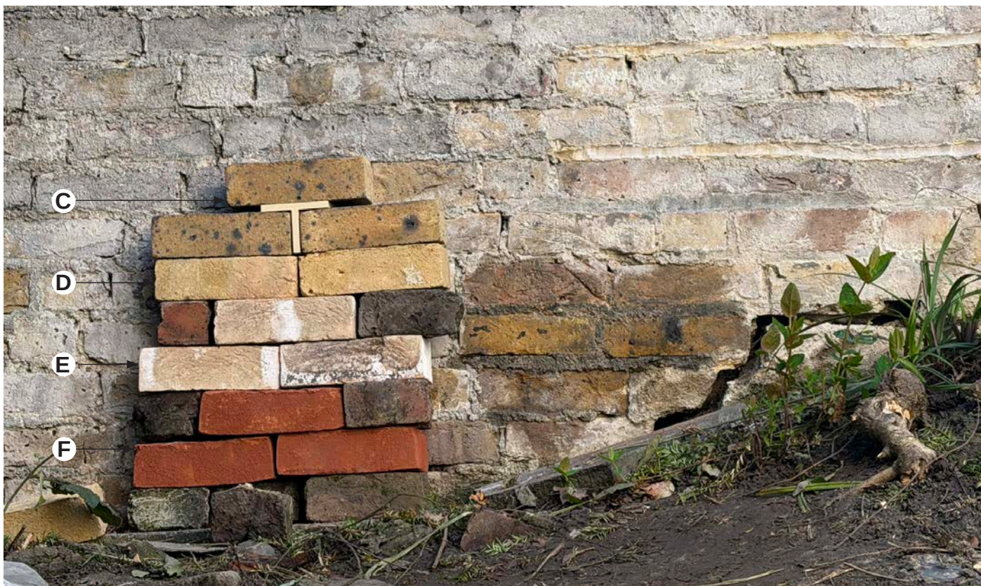
Photograph F - Closeup of Shortlisted bricks also showing a wetted section of the existing wall to remove efflorescence.
