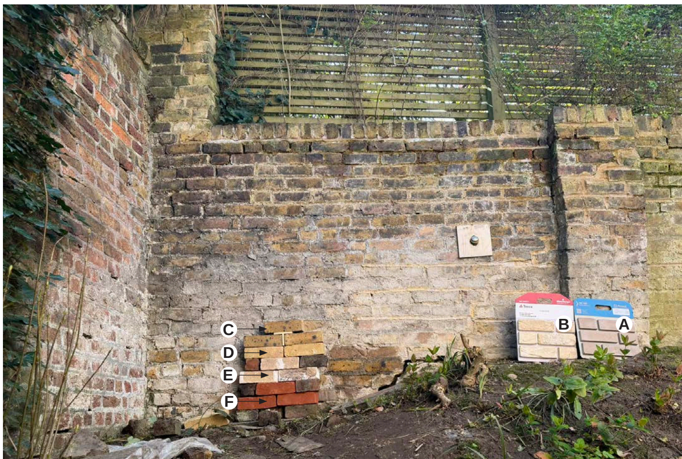
Photograph D – Cleaned section of existing boundary wall in a dry state.
