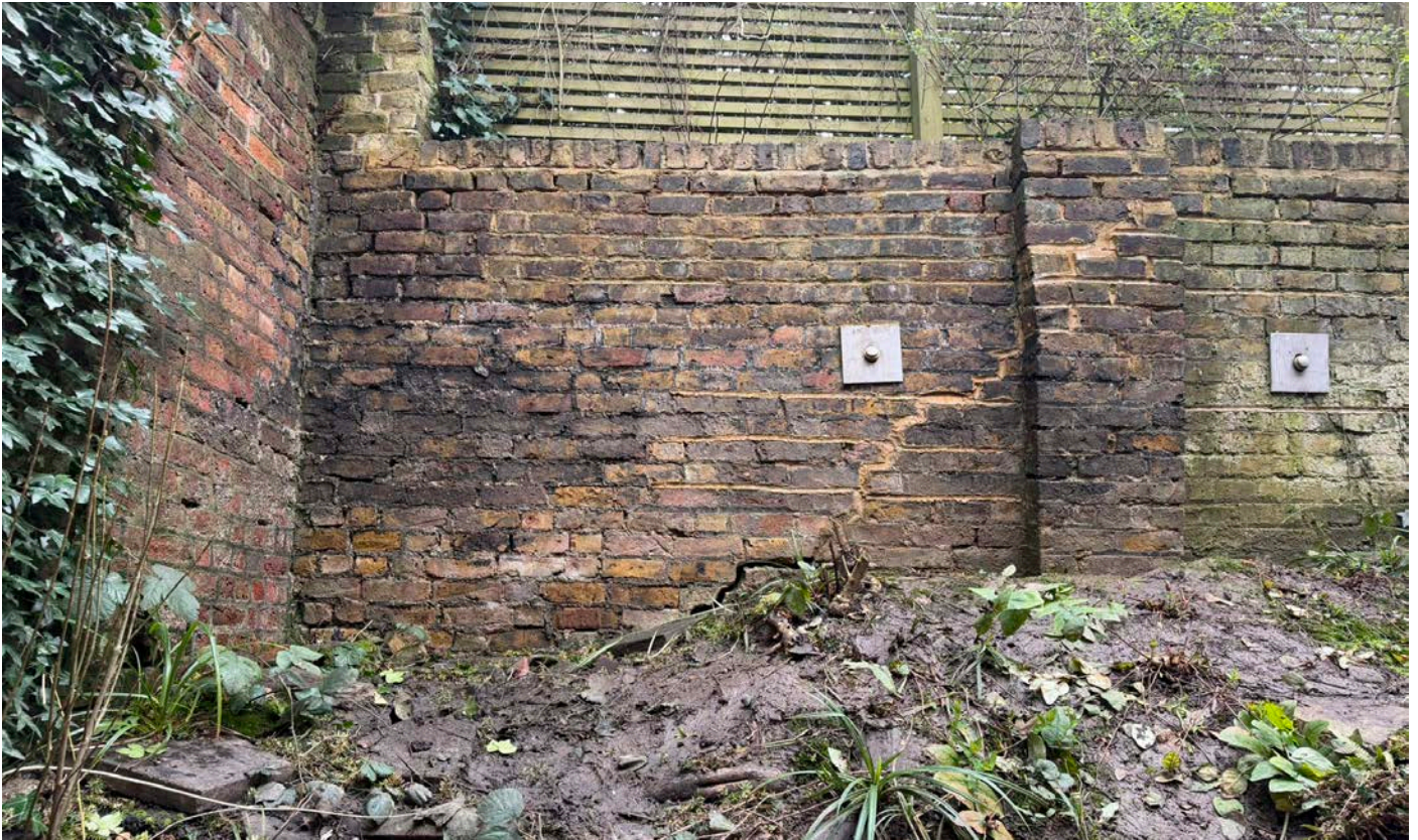
Photograph B - Cleaned section of existing boundary wall in a wet state.
