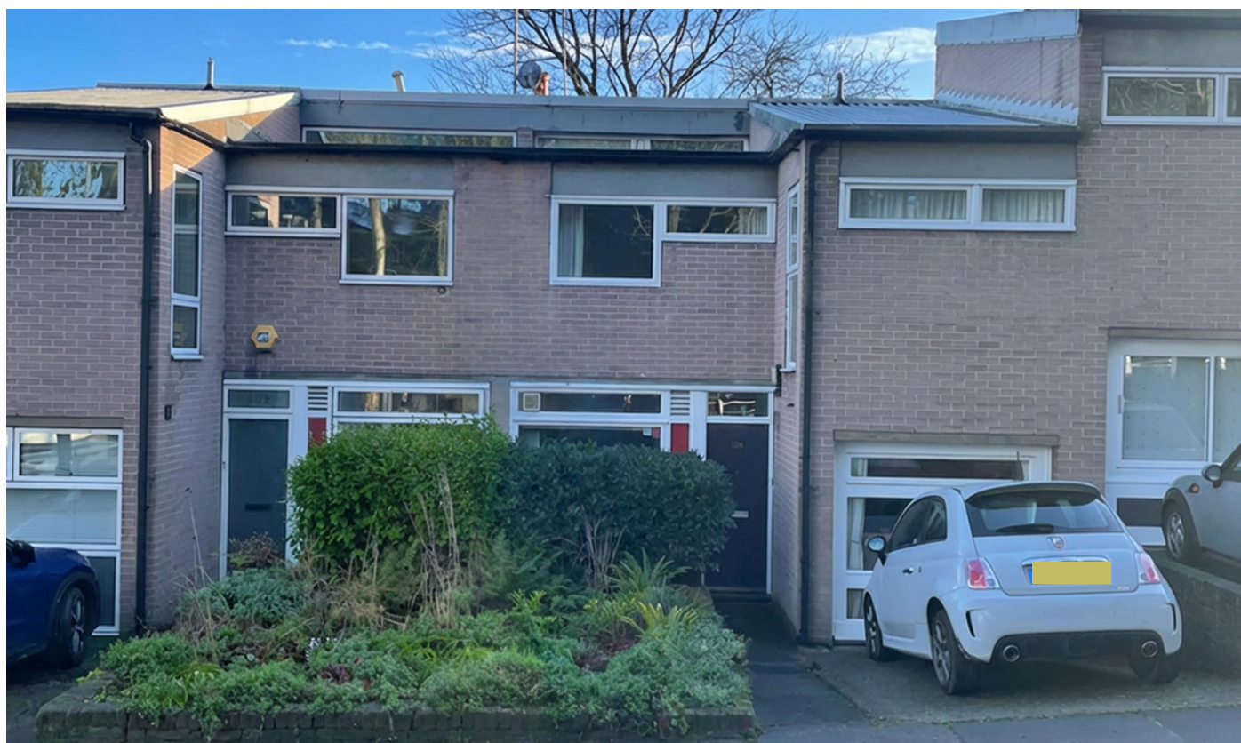
No. 106 Southwood Lane Timber window material, no glazing bars, flush profile, white colour.
