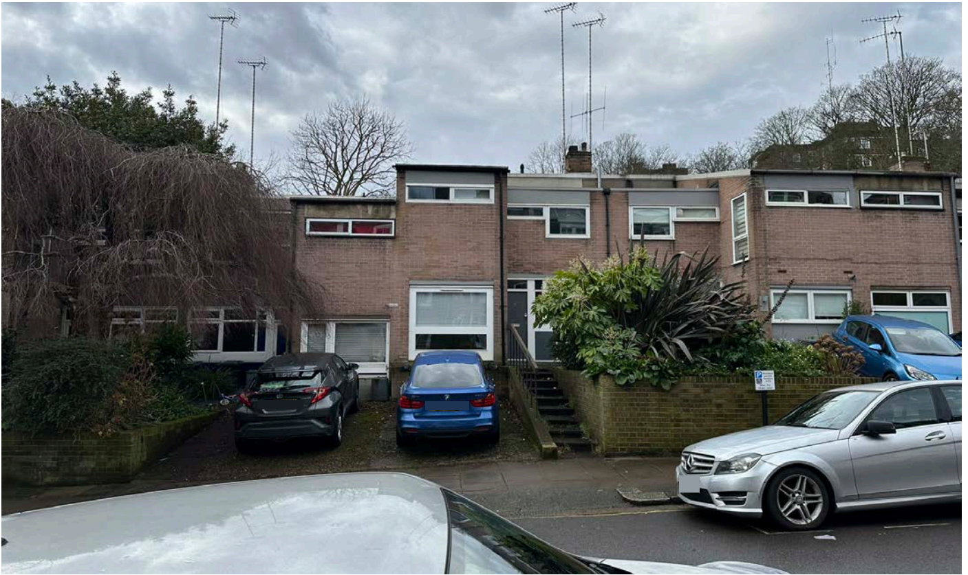
No. 9 and 11 Hillside Gardens Appear to be uPVC (11) and Timber (9) Window material, no glazing bars, flush profile, white colour.
