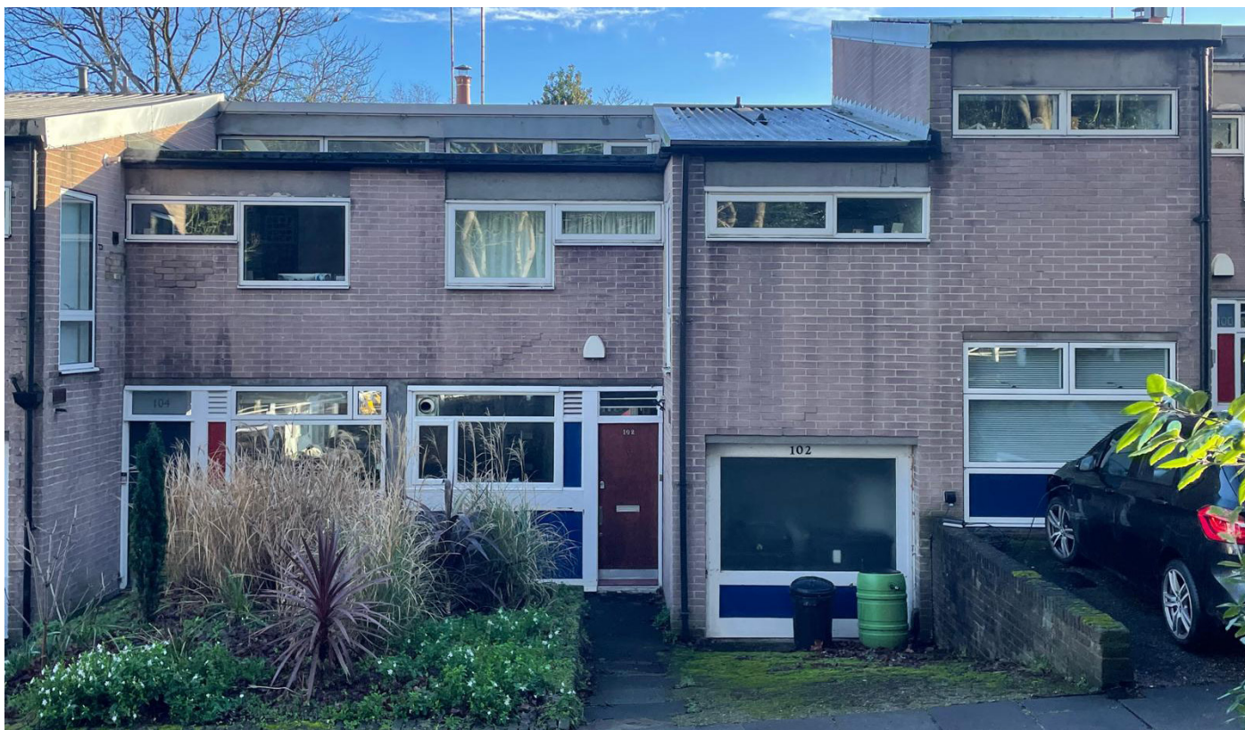
No. 102 Southwood Lane Appears to be uPVC, no glazing bars, flush profile, white colour. No. 104 Southwood Lane Appears to be Aluminium (likely Velfac, Idealcombi or similar), no glazing bars, flush profile, white colour.
