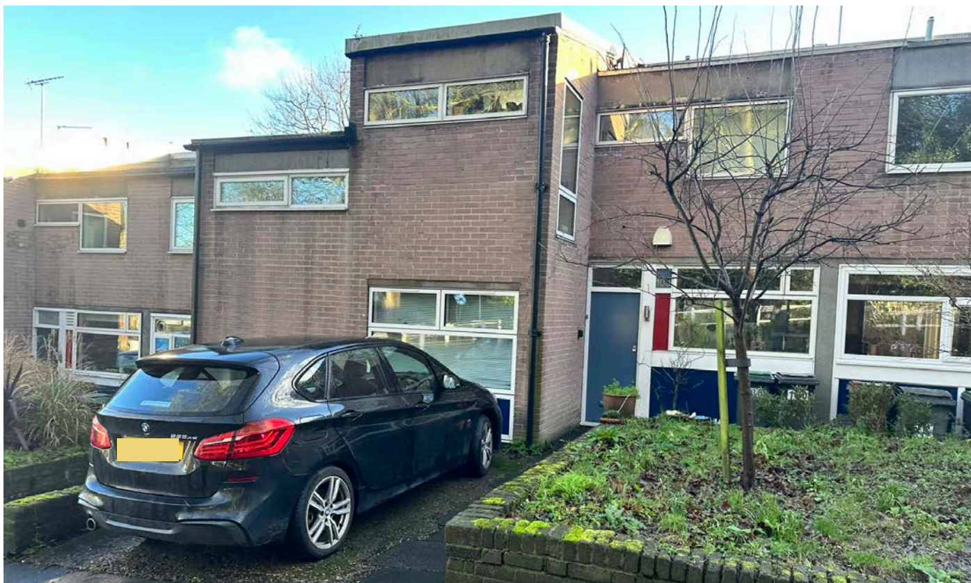
No. 100 Southwood Lane Aluminium windows (likely Idealcombi, Velfac or similar), no glazing bars, flush profile, white colour. Garage detailing is a significant departure from the 1958 design.
