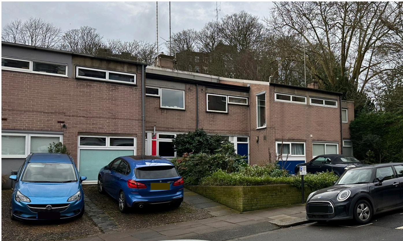
1, 3 & 5 Hillside Gardens, Appear to be a mix of uPVC, aluminium and Timber Window material, no glazing bars, white colour. Garage detailing and some windows are a significant departure from the 1958 design.
