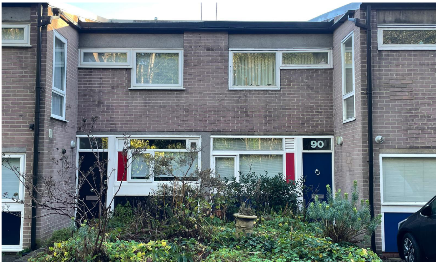
No. 90 Southwood Lane Timber window material, no glazing bars, flush profile, white colour. No. 92 Southwood Lane UPVC window material, no glazing bars, white colour. Garage detailing is a significant departure from the 1958 design in both properties.
