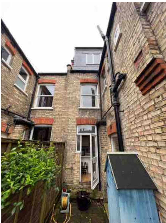
External - Rear Side alley - Location of proposed extension
