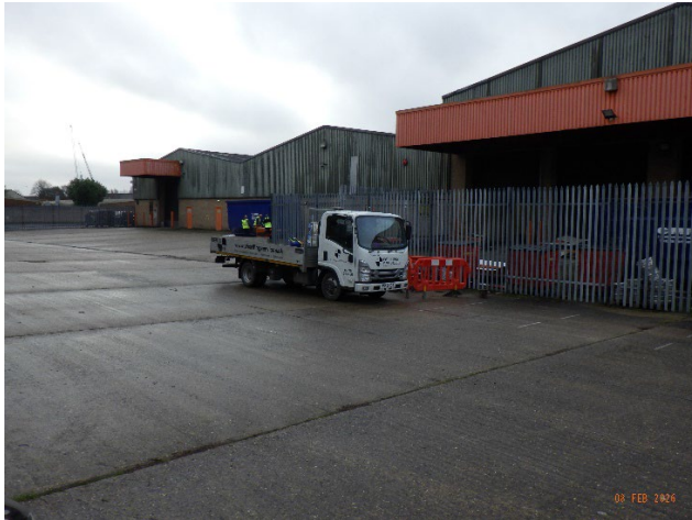
Photo 1 Secure working area over BH01
