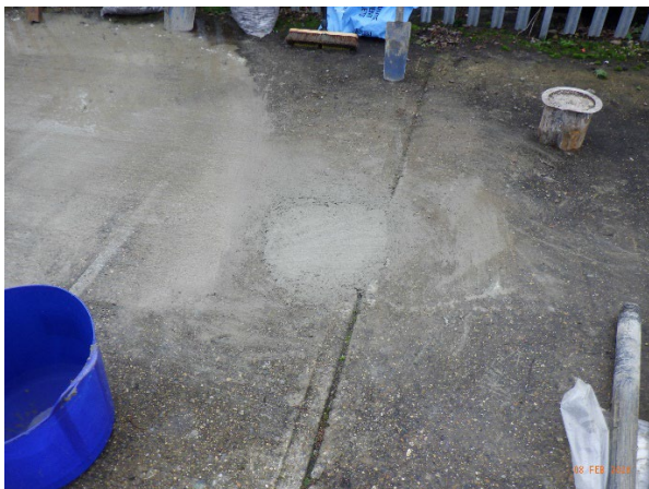
Photo 5 BH01 Surface concreted and finished over bentonite seal
