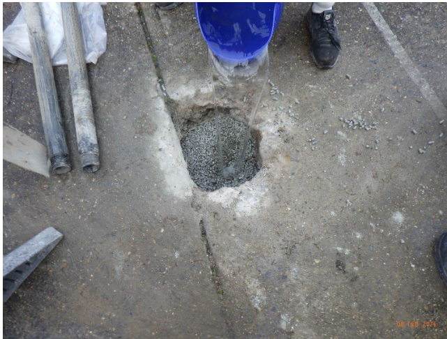
Photo 4 BH01 Final bentonite placement at top of well following backfill
