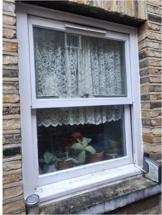
Rear Side Ground Floor Window
