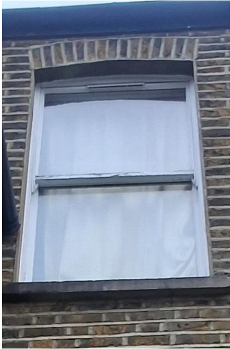
Rear First Floor Window
