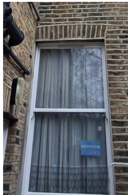
Rear Ground Floor Window
