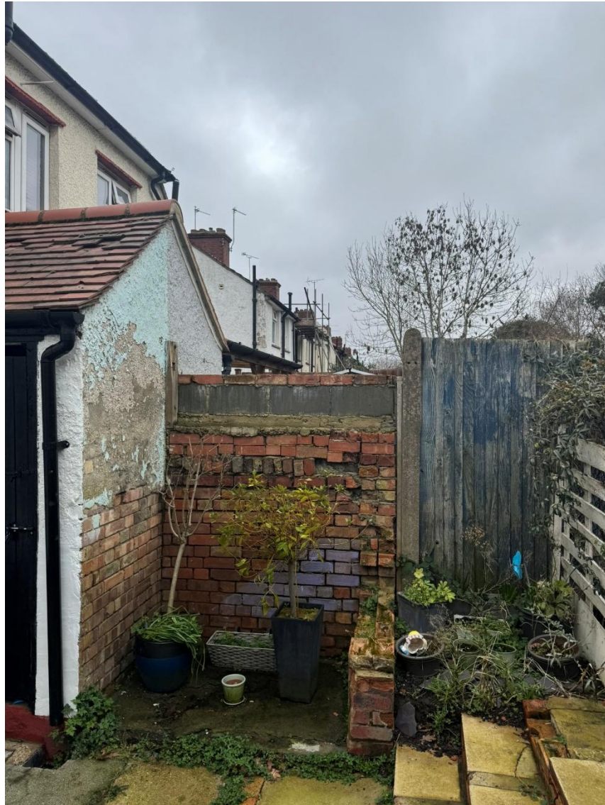
Fig 8. View looking towards boundary with no.27 showing existing outbuilding/coal shed and boundary features
