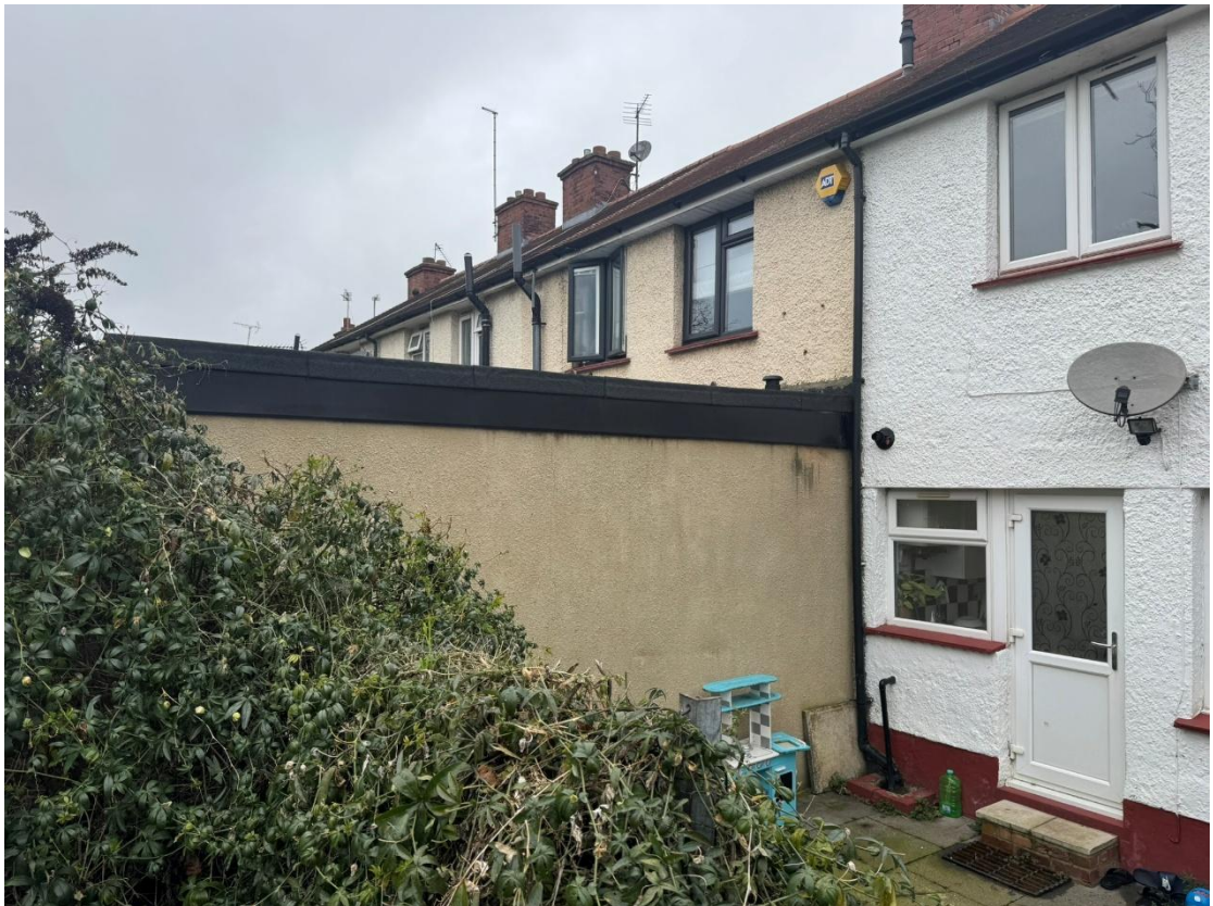
Fig 7. Rear view looking towards no.29 showing 5m deep neighbouring extension
