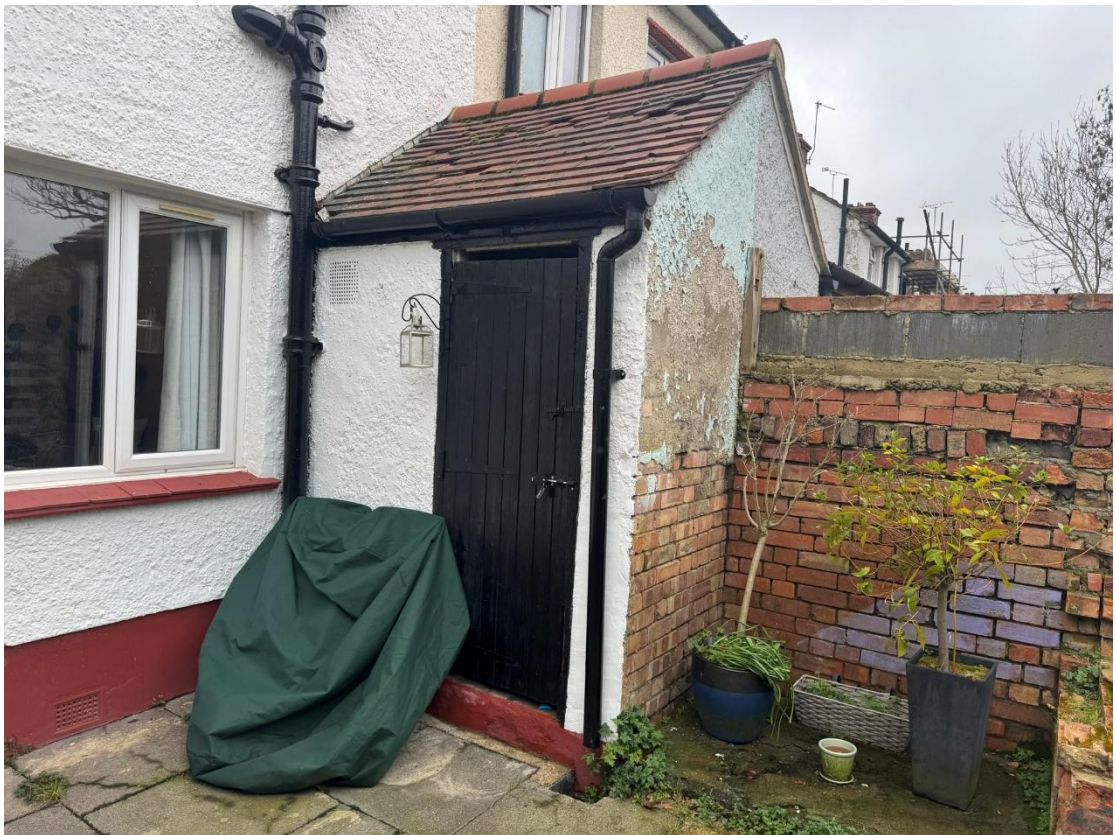
Fig 8. Rear view looking towards no.27 showing existing outbuilding/coat shed
