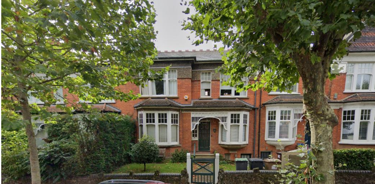
Figure 1. 5 Firs Avenue Road, Front Elevation (Google Maps, September.2025)
