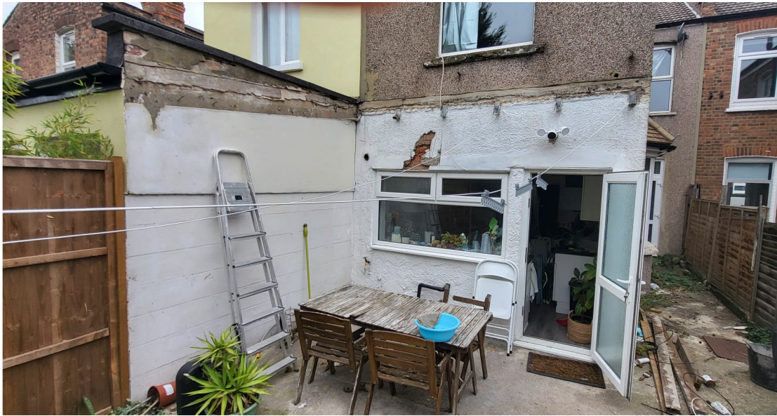
View of rear patio area
