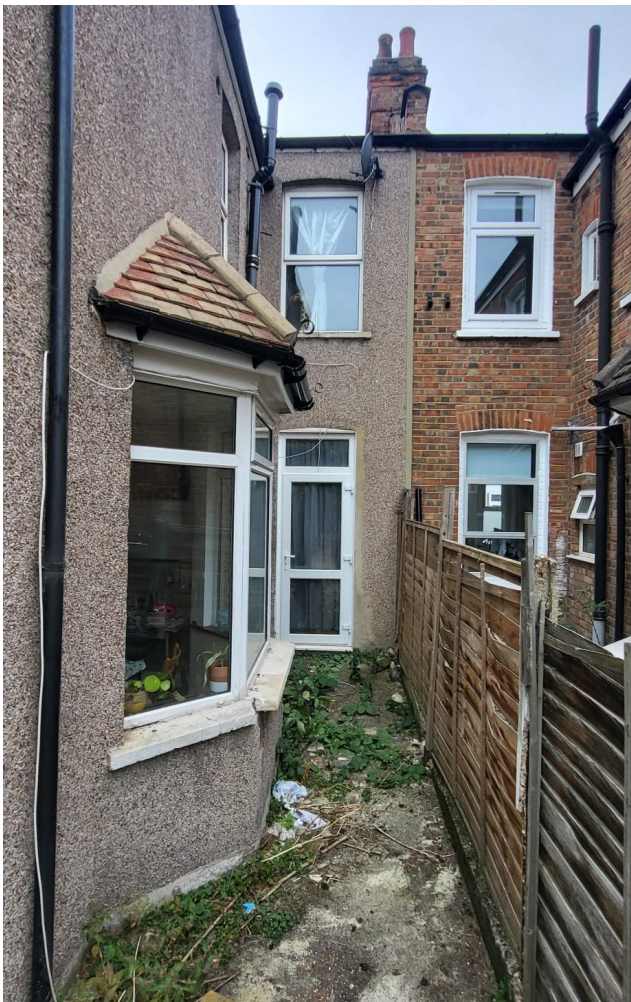
View of side infill area
