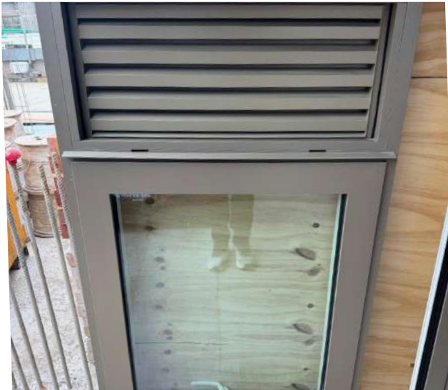
PRODUCT NAME: INWARD & OUTWARD OPENING ALUMINUM WINDOWS IN RAL 1035 (WITH LOUVRE) MANUFACTURER: ALURON ITEM NO. IN SAMPLES TRACKER: 5.02
