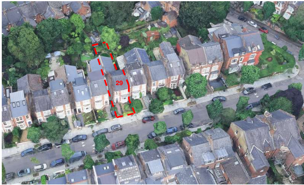
Front bird's-eye view of the house
