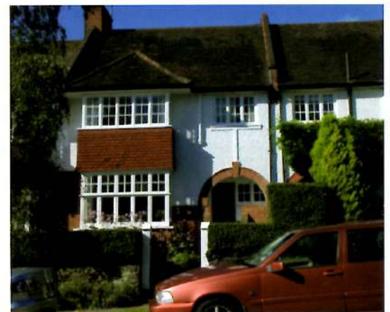
Fig. 3.9 Rookfield Avenue Stage 2. Type D.
