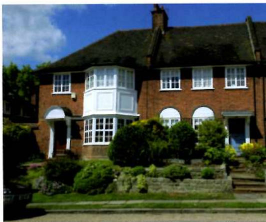
Fig. 3.20 Part of 1 to 29 Cascade Avenue.
