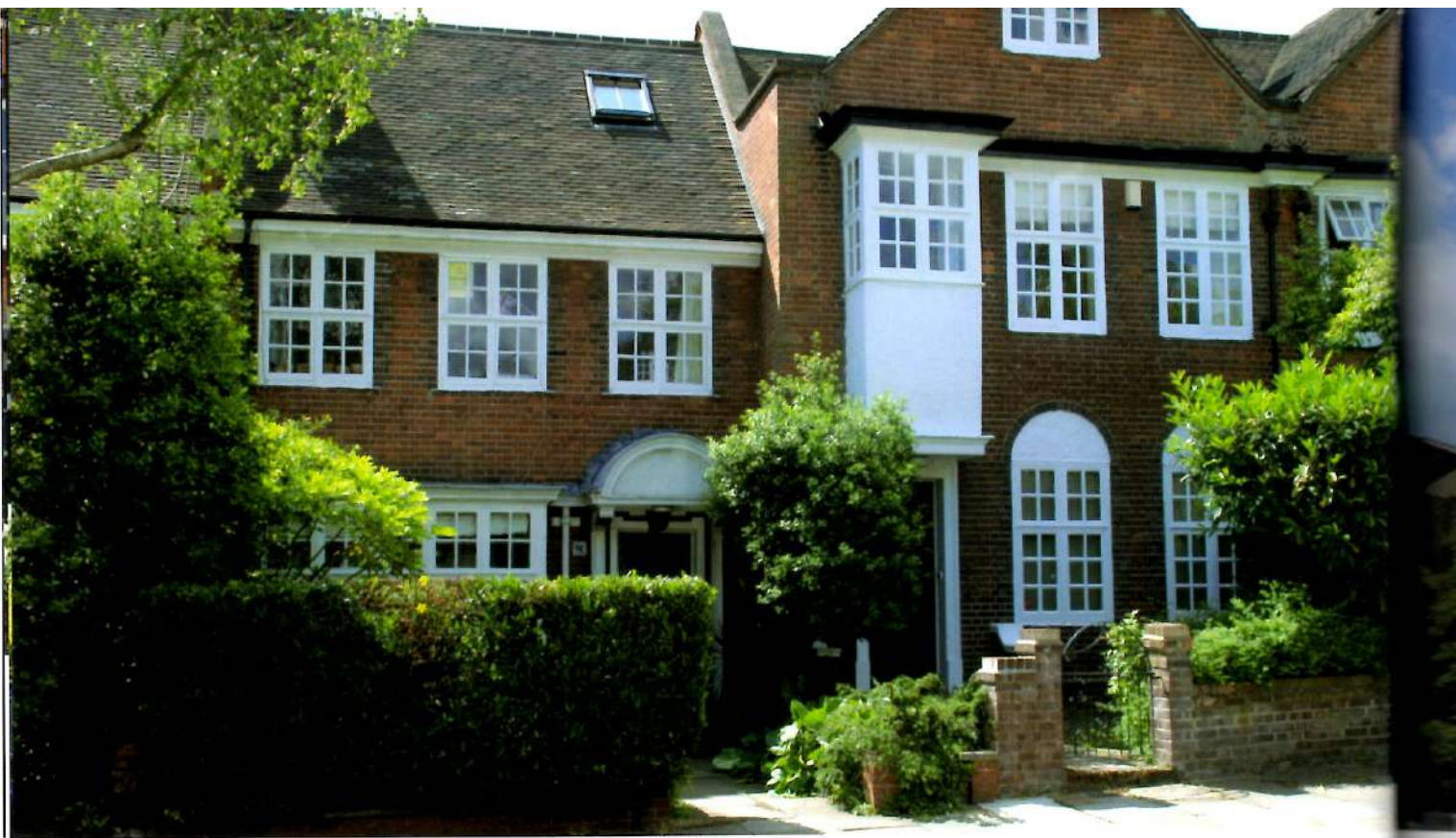
Fig. 3.19 Etheldene Avenue 74 to 88. Approved 1911. The first time that W B Collins had designed a half-hipped gable.
