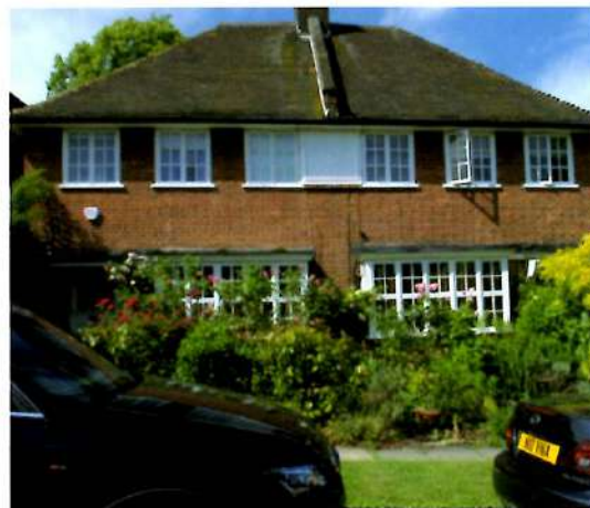
Fig. 3.26 55 & 57 The Chine 1913, the last houses built with party walls projecting above the roof.
