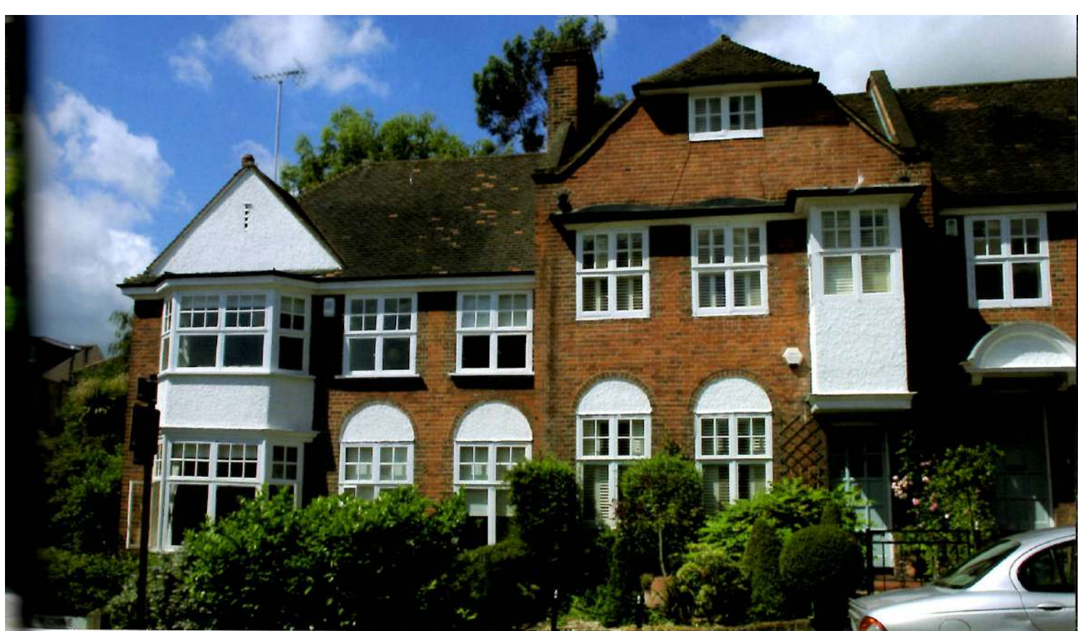
Fig. 3.22 The Chine 1 to 11 approved 1911, showing a half-hipped gable.
