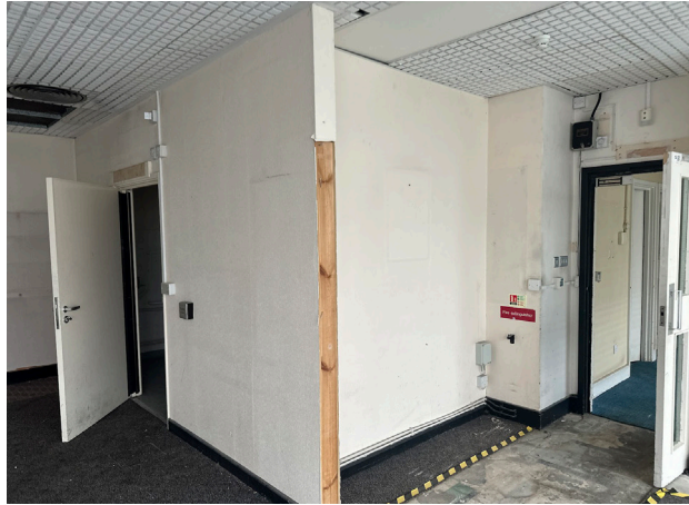
Plate 15 View of modern partitions and suspended ceiling to east of the building.
