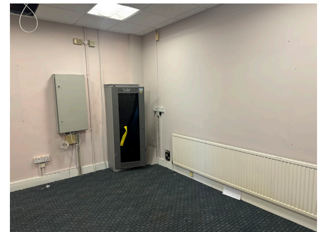
Plate 28 Modern floor and partition to mezzanine level.
