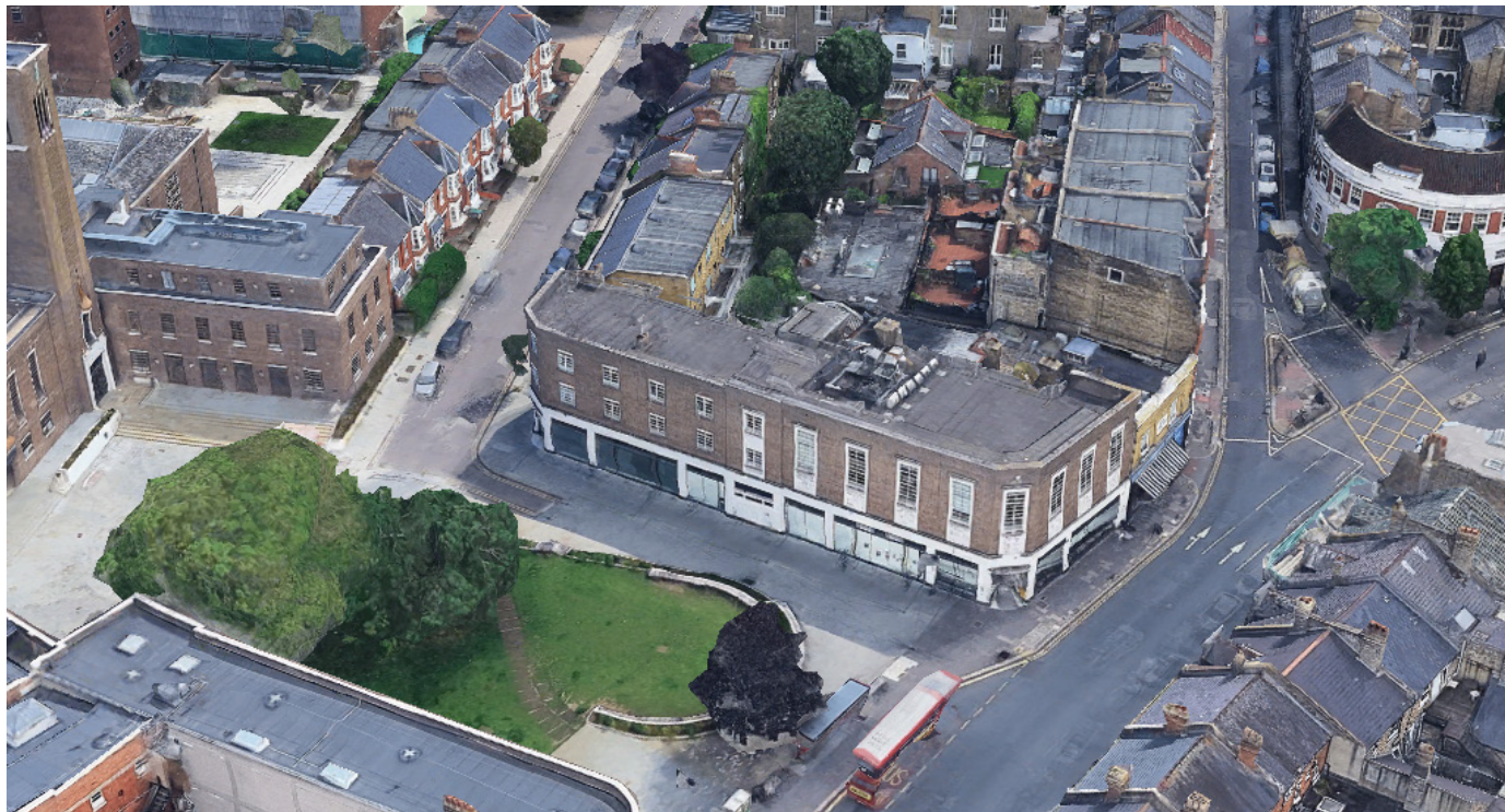
Figure 12 Oblique aerial mapping looking southeast showing the site (1) and section of the conservation area (whole image-2). Other heritage assets are visible in this image but due to the limited nature of the works are not considered to be affected by the proposals.
