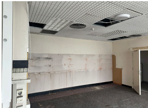
Plate 17 showing historic south wall and modern partition to right.
