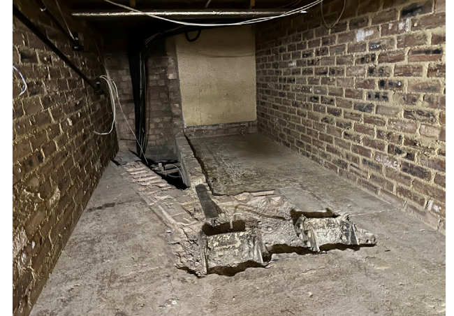
Plate 31 Likely historic steel and brick foundations of former stage at first floor.
