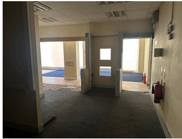
Plate 7 Looking north across the entrance room showing modern partitions and suspended ceilings.
