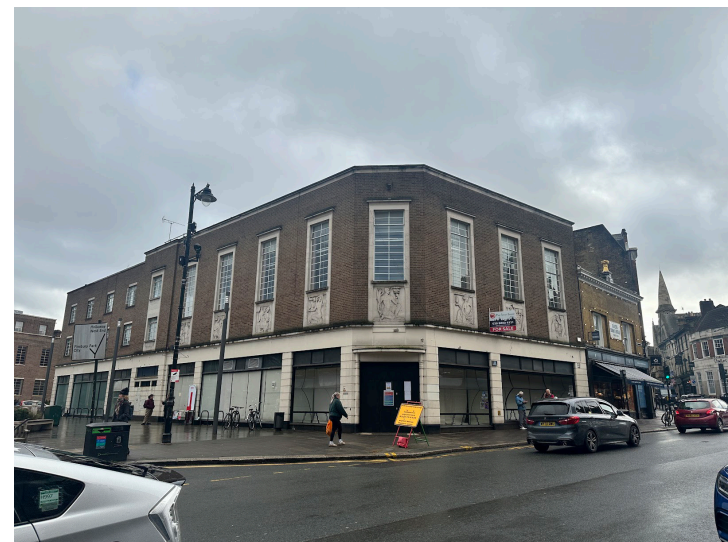
Plate 2 View looking southeast towards west and northern elevation of the site.
