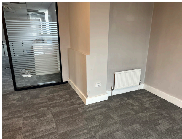
Plate 27 Modern floor and partition to mezzanine level. The floor is roughly on the line of the original office above the demonstration room.
