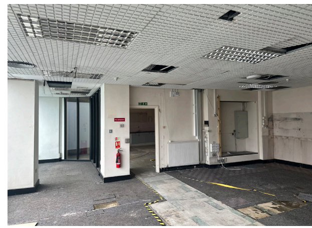
Plate 18 View eastern towards eastern end of the building showing historic piers and potentially historic concrete floor with green and black inlay.
