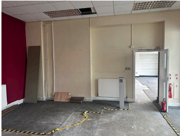
Plate 19 View west from easternmost room. Part of the wall is likely original with modern stud infil.
