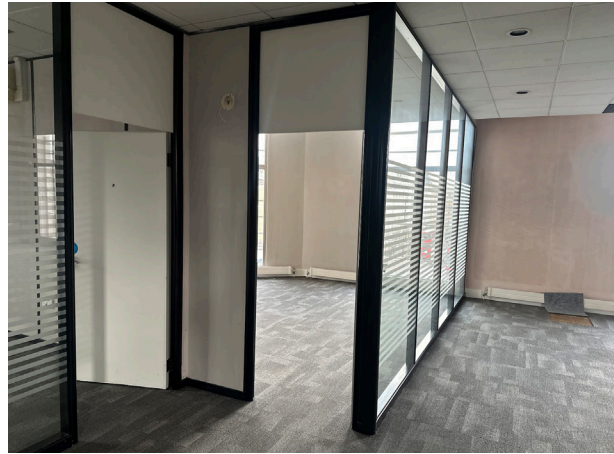
Plate 24 Modern floor and partition to mezzanine level.
