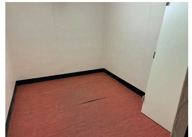
Plate 34 Small rear room to eastern end of first floor. Appears to be historic dimensions but no original fixtures or fittings surviving.
