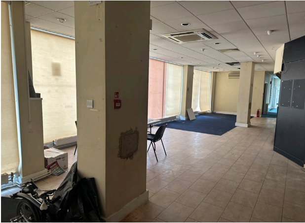
Plate 3 View looking north east from the entrance in the former show room. The piers are historic, the partition on the right modern. Note modern suspended ceiling also.
