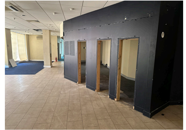
Plate 5 View of modern partition in historically open space.
