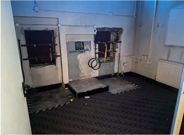
Plate 9 Side room to the northern side of the building with later ATM openings. No historic fixtures or fittings visible.
