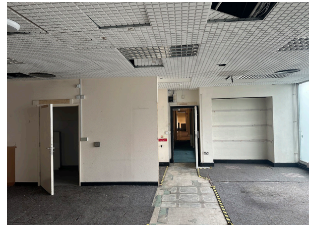
Plate 16 view west from eastern part of the building. Remnants of historic wall visible to the right with modern partition to the left.
