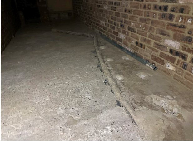
Plate 29 Historic concrete floor and modern brick piers at first floor beneath the mezzanine level. The curved in the concrete potentially corresponds with the seating seen in the historic plans.
