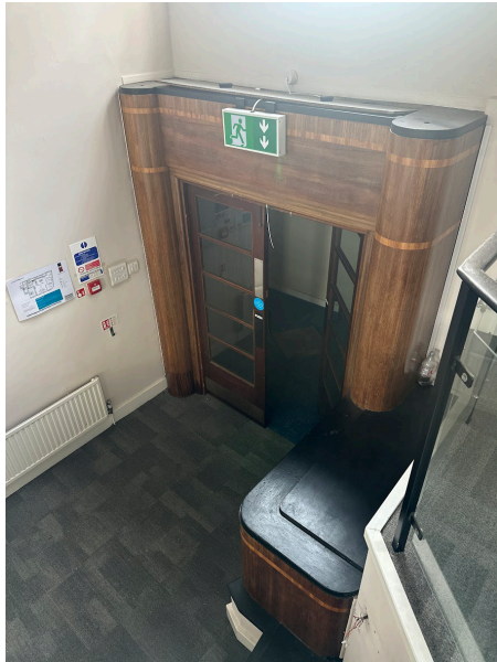
Plate 23 View of original timber door surround to first floor from mezzanine level.
