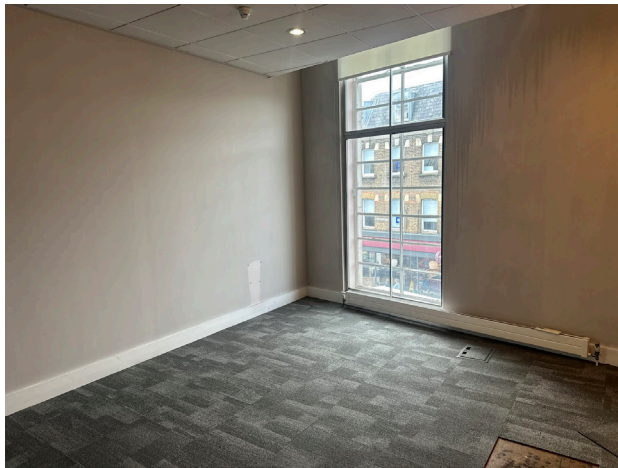
Plate 26 Modern floor and partition to mezzanine level. The floor is roughly on the line of the original office above the demonstration room.
