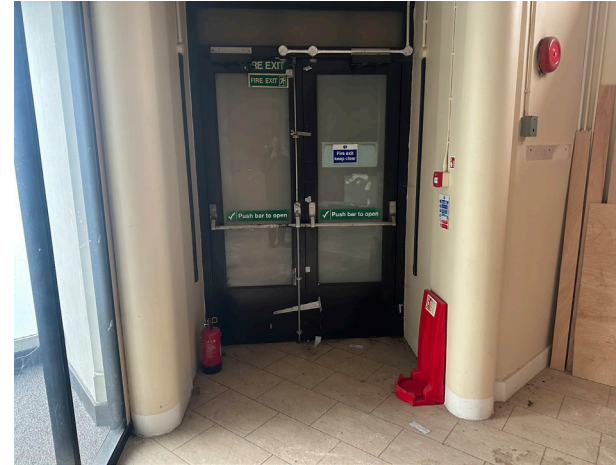
Plate 20 View of secondary entrance to north eastern corner with Art Deco curved surrounds.
