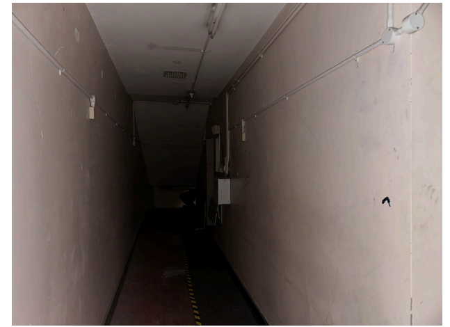
Plate 8 Corridor to the south of the building showing original room proportions but no visible historic fixtures or fittings.
