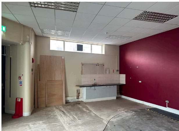
Plate 21 View of easternmost room showing historic entrance door surround (left) and no other visible fabric of interest.
