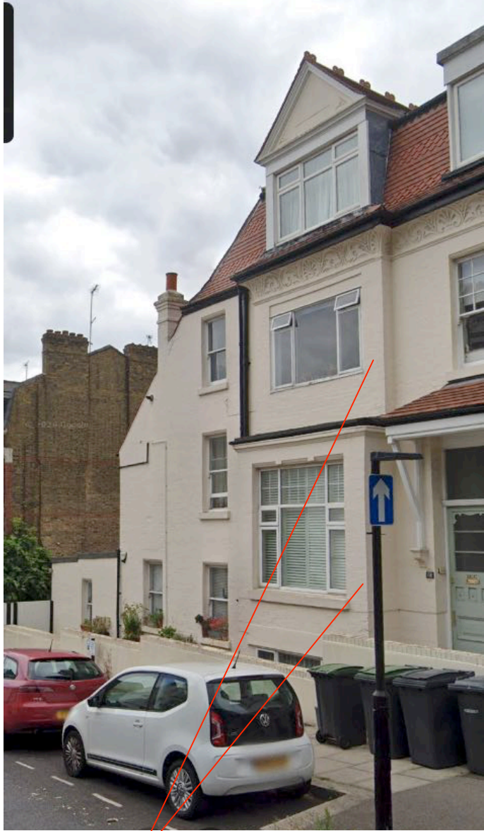
Existing side showing bays modulating the facade
