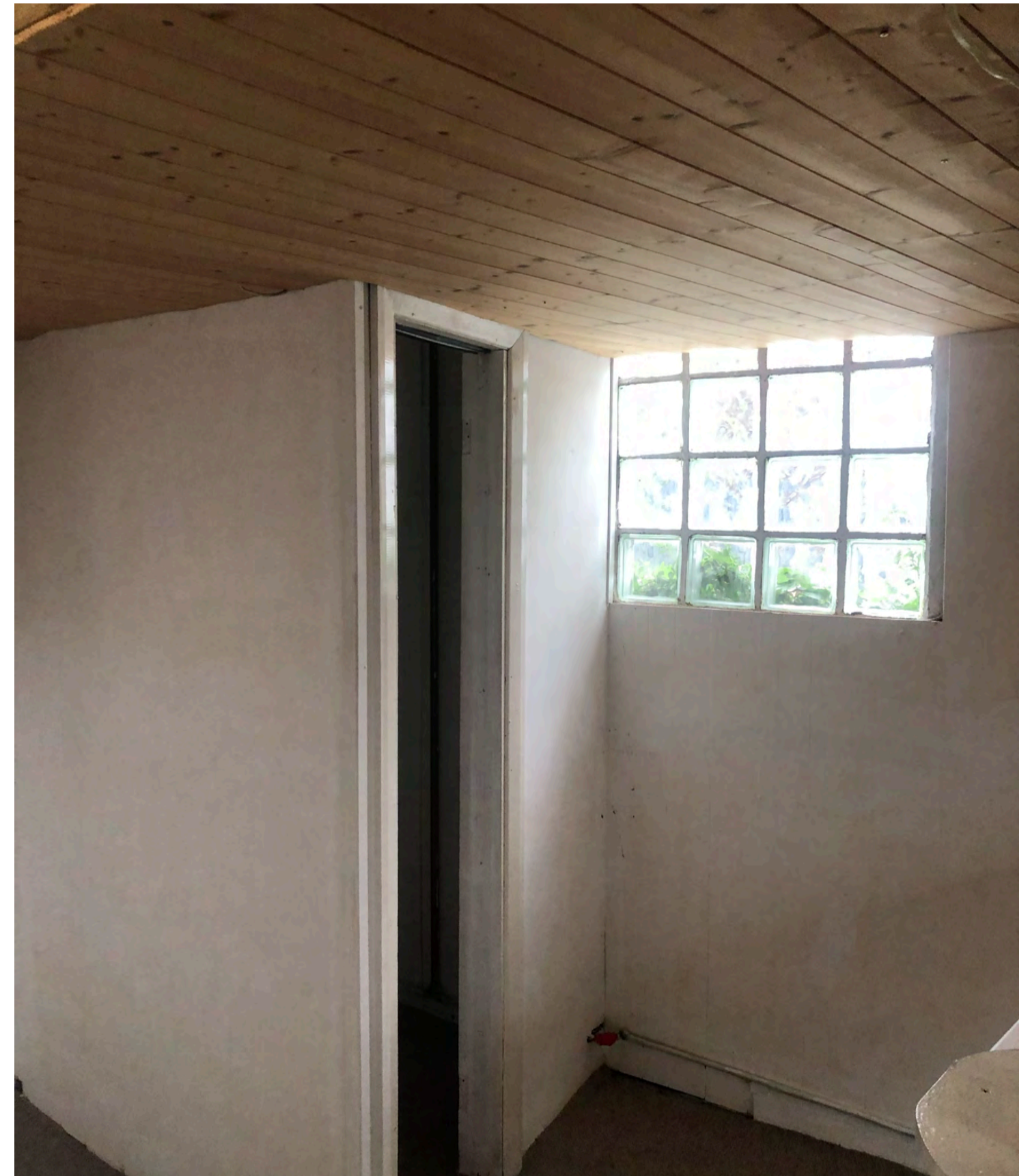
Internal view looking west at boundary wall which fronts the garden of number 110 Nelson Road
