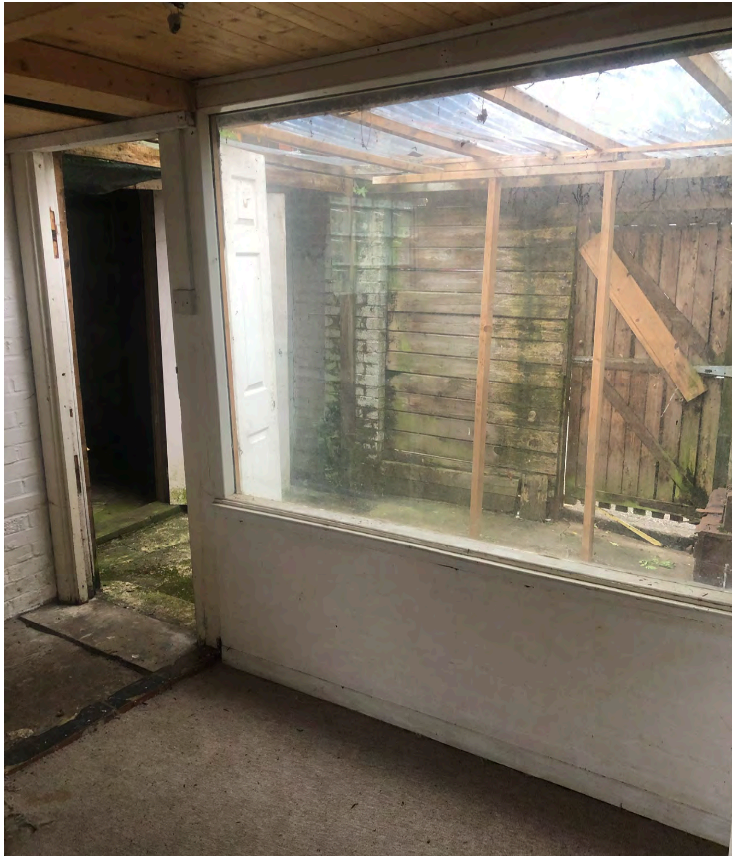
Internal view looking north at the internal wall leading out the entrance yard and Weston Park Road beyond
