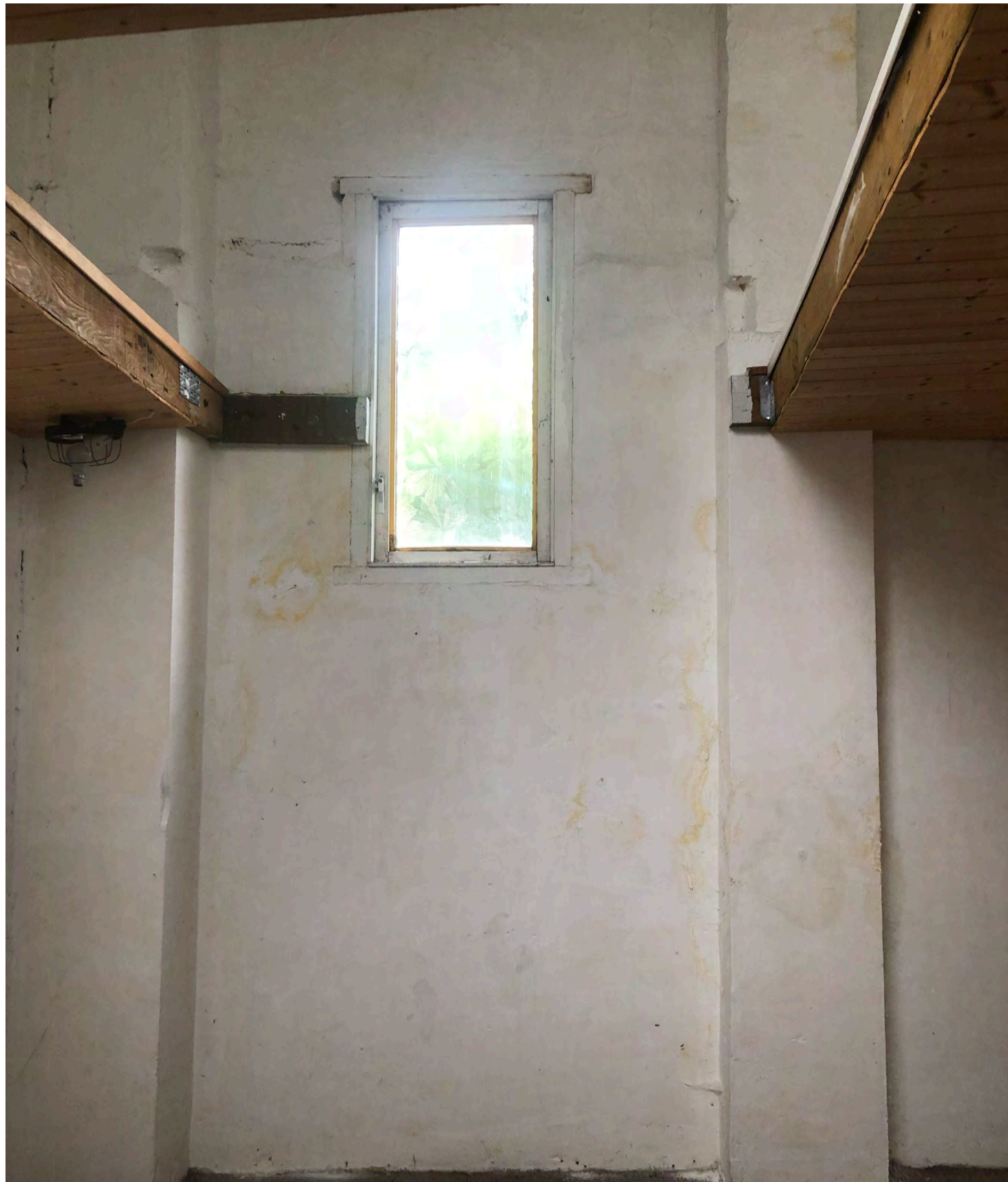
Internal view looking south at boundary wall which fronts the garden at number 108 Nelson Road
