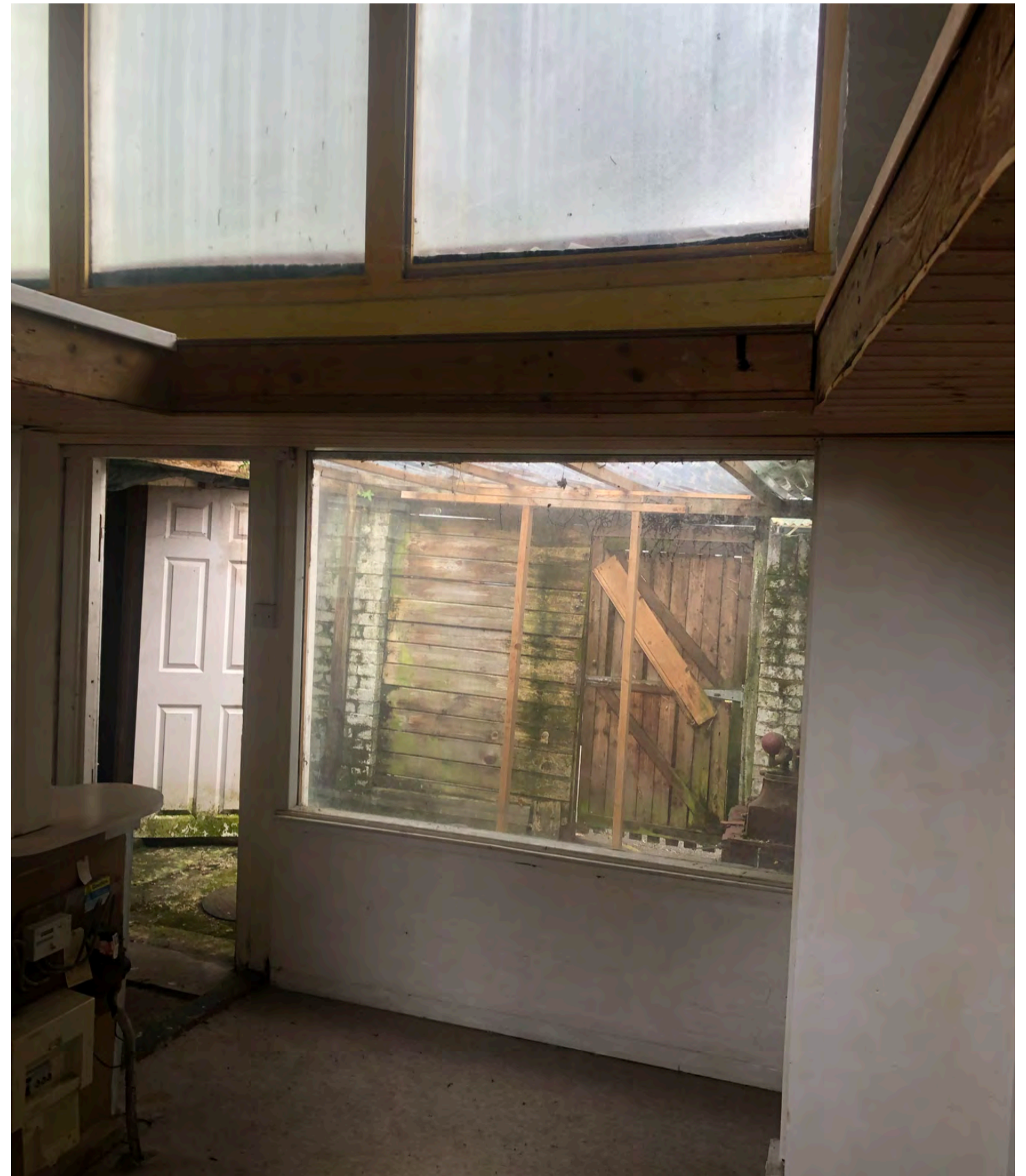
Internal view looking north at the internal wall leading out the entrance yard and Weston Park Road beyond. Clerestory windows above.
