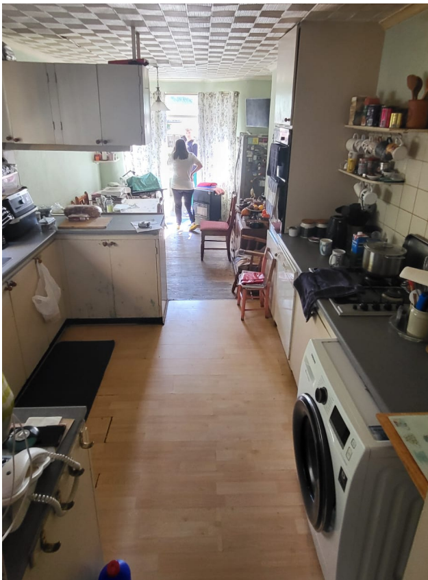
Internal views of existing Kitchen/Dining room
