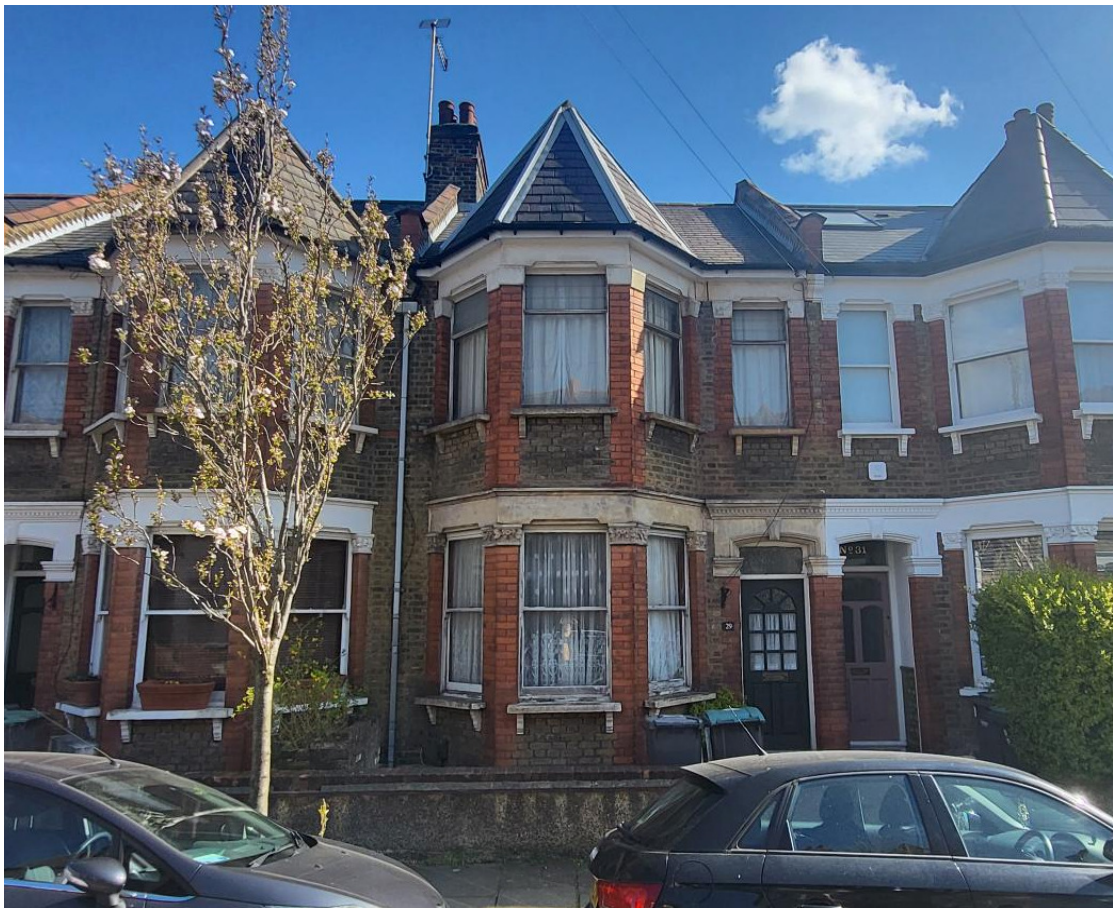
Front elevation view of the property
