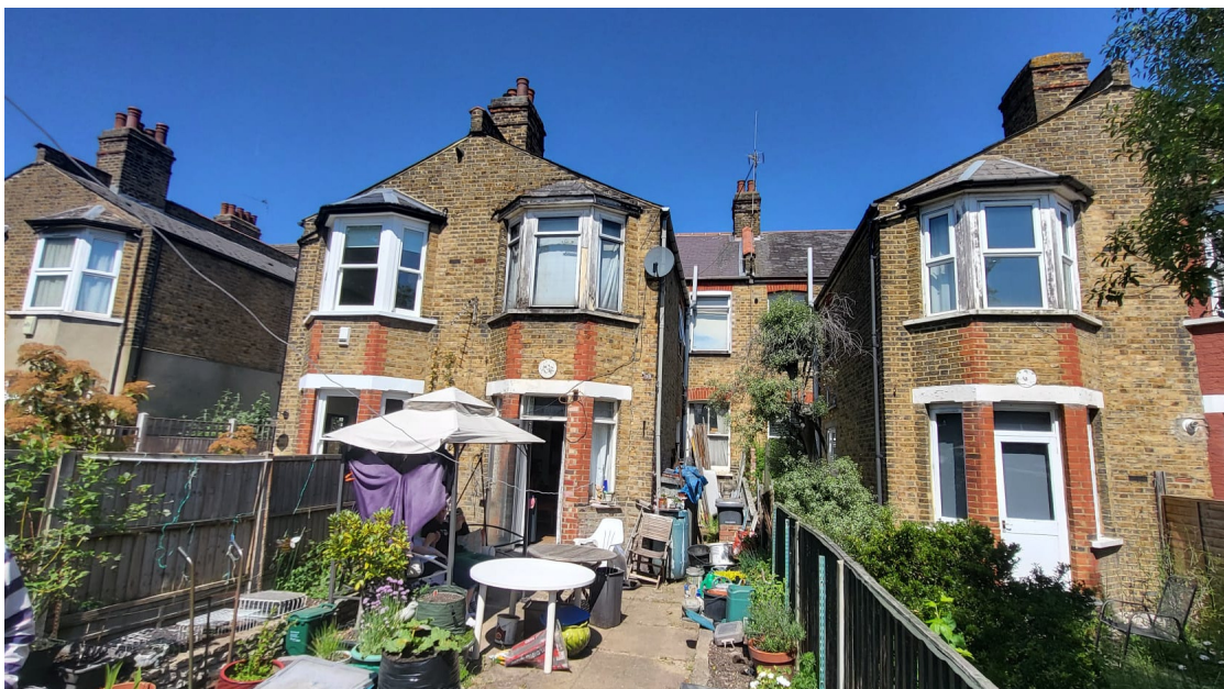
Rear elevation view of the property
