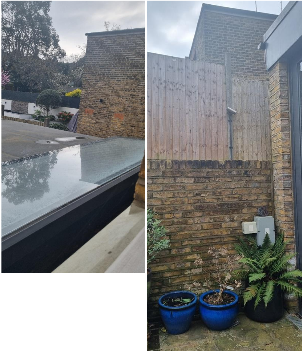
Photo 2 – Boundary condition and existing enclosure
