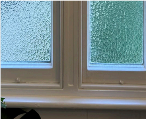
Latch fixings operable with external latches
