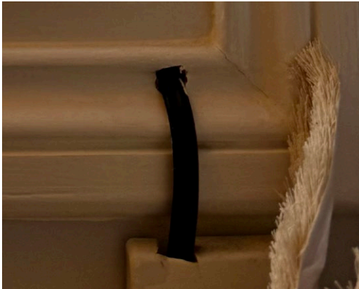
Hole in frame made for cable
