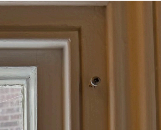
Screw drilled into frame
