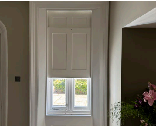
Vertical shutters operable with visible rope pulley system
