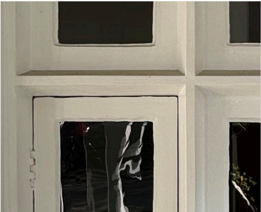
Not fully sealed when closed
