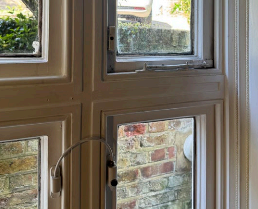
Modern locking system, window stay for top right casement not operable
