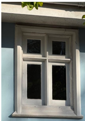
WFF.01 (FRONT) Stair Good internal and external condition
