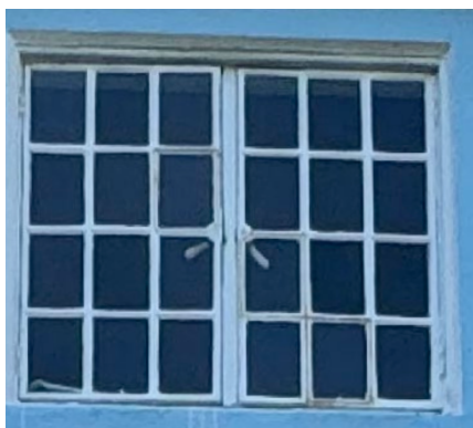
WFF.03 (REAR) First Floor Bedroom
