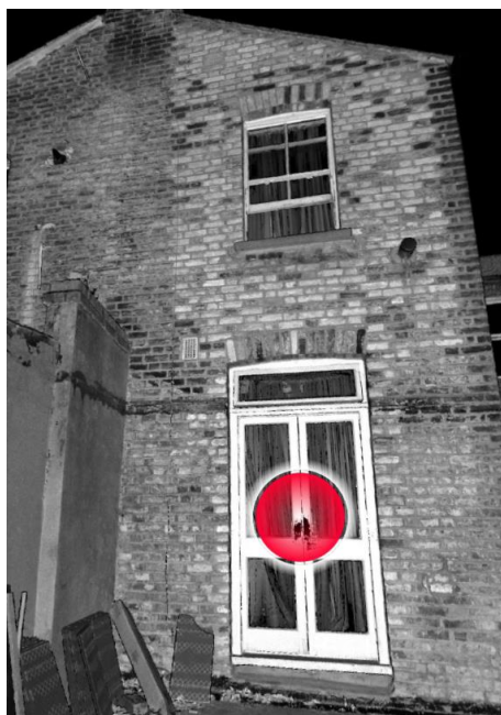
Rear End Elevation Exit Doors
