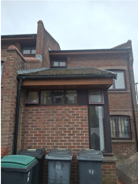
Front Ground Floor Communal Entrance Windows
