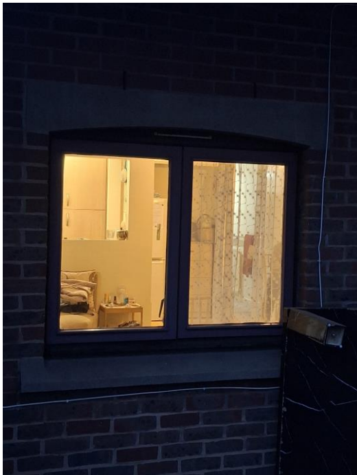
Rear Ground Floor Window
