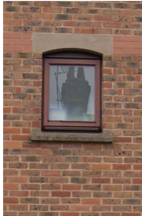
Side First Floor Window
