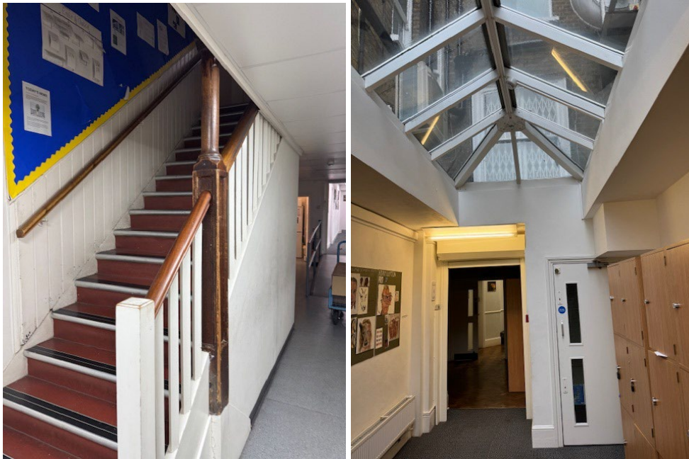
Lower Ground Staircase and Ground Floor entrance to staircase
