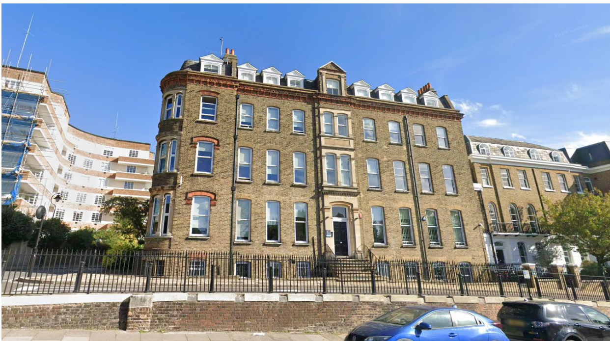
Channing School (Centre) – Slingley and Westview to the right, Cholmeley Lodge to the left
