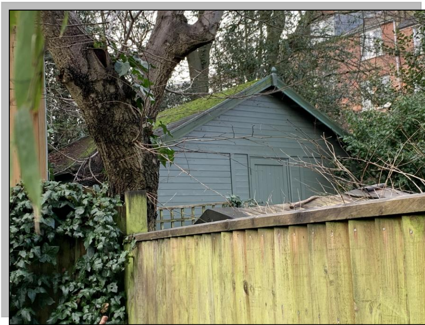
Photograph of outbuilding in rear garden of Jacksons Lane to rear of 34 Southwood Avenue.
