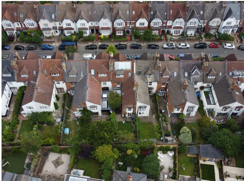
The property at no.11 Berkeley Road shown from the rear
