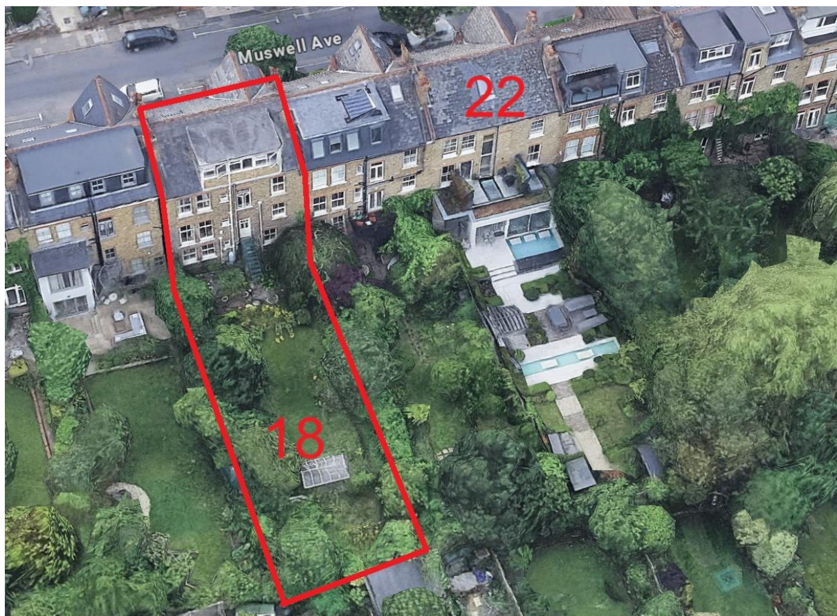
AERIAL VIEW SHOWING SIMILAR EXTENSION AT NO 22 MUSWELL AVENUE
