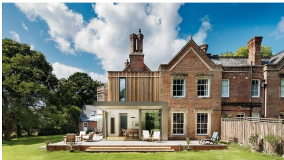
Cedar timber addition to listed Georgian Vicarage. Hampshire
