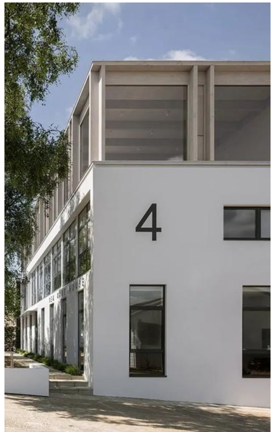
Douglas fir framed roof extension to light industrial building NW2.
