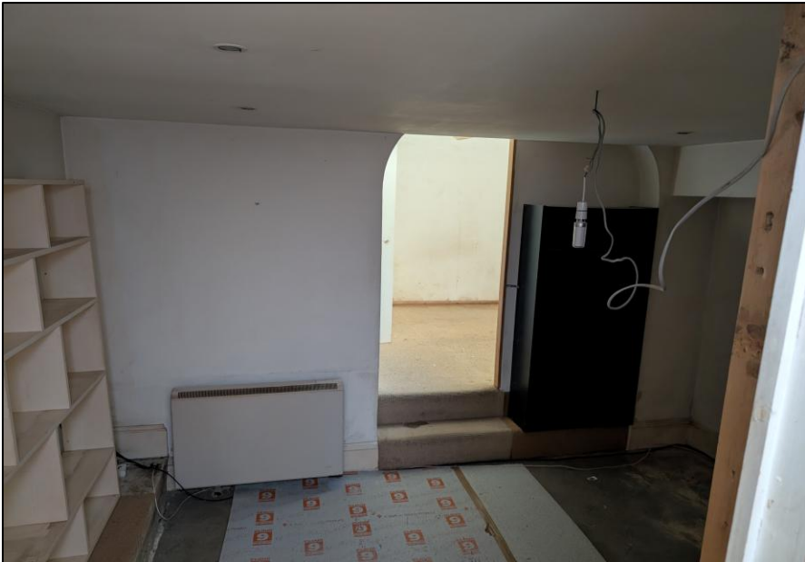
Figure 16: Lower Level Interior
