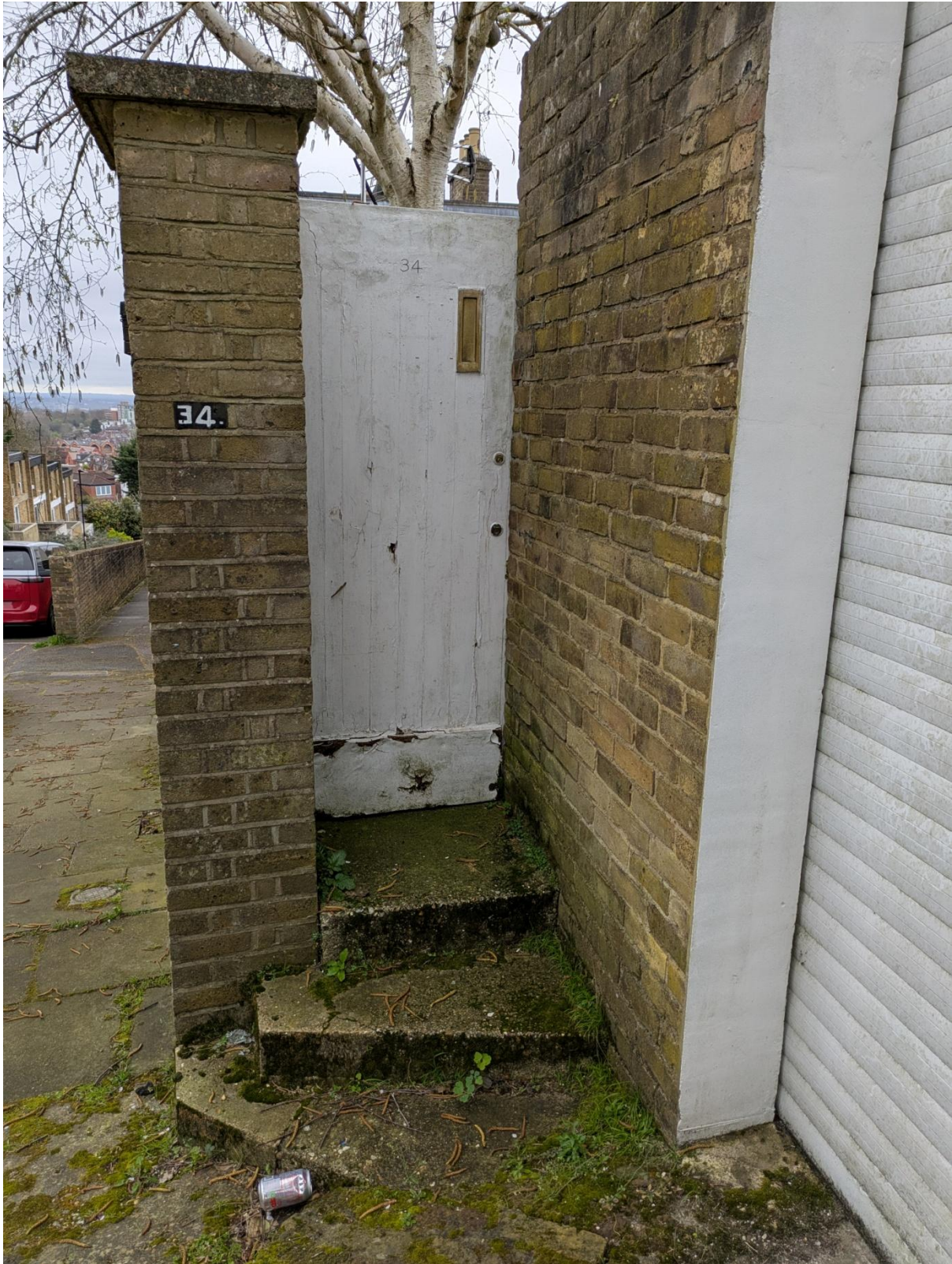
Kingsley Place narrow gated stepped entrance
