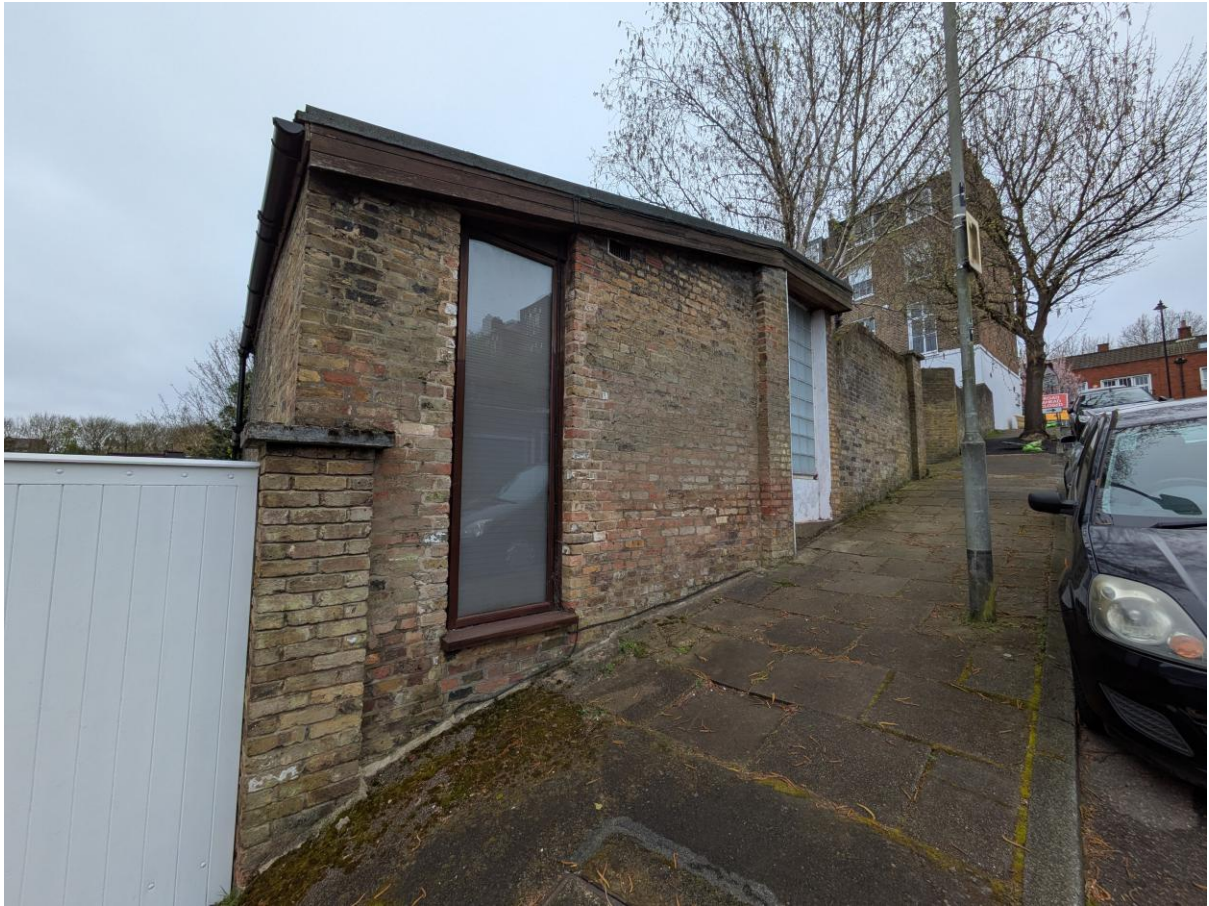
34 Kingsley Place east end
