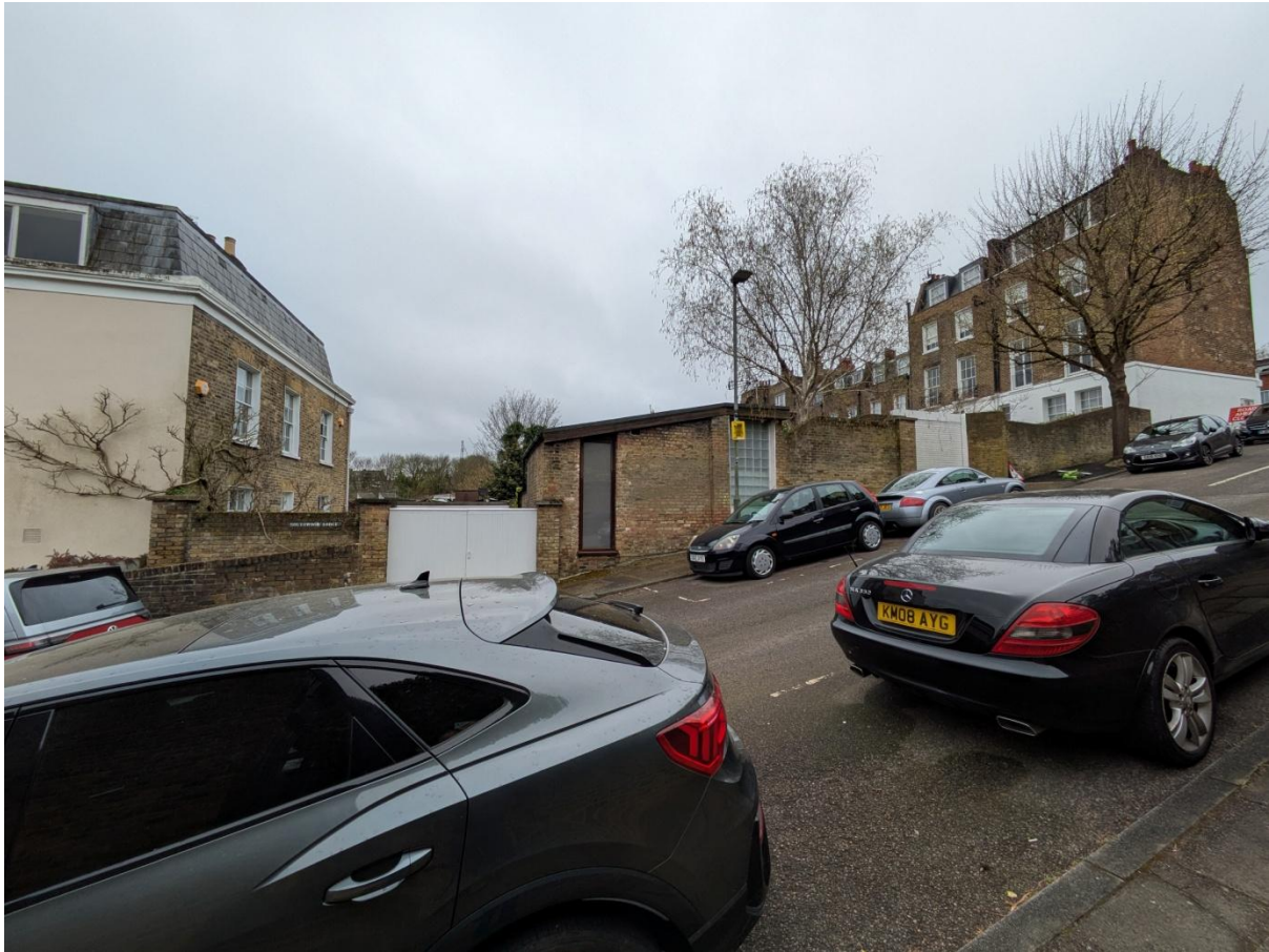
Kingsley Place view overall south
