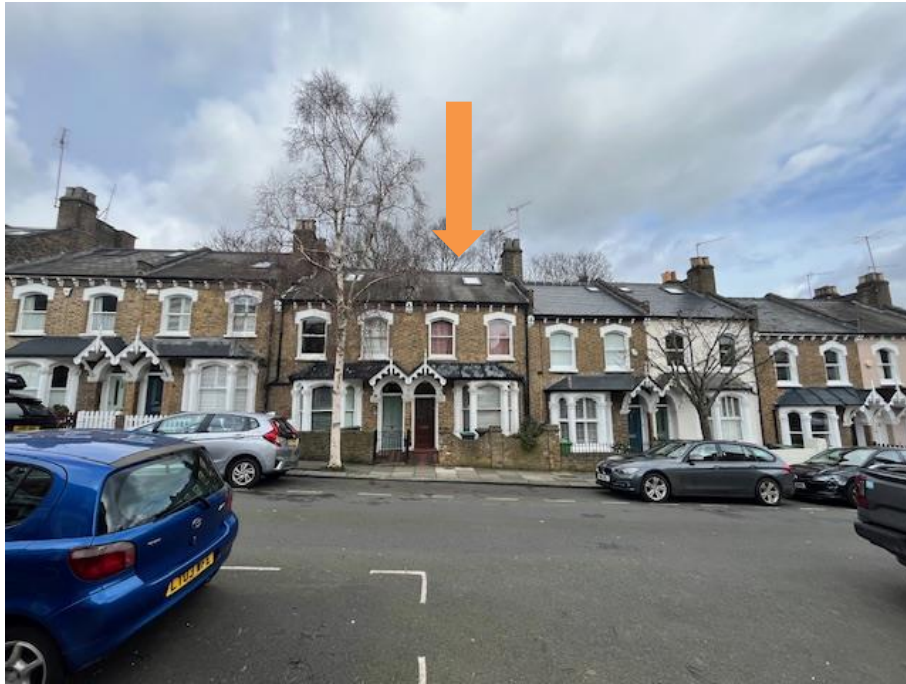
Photo 2 – Front Elevation in relation to other properties on the street
