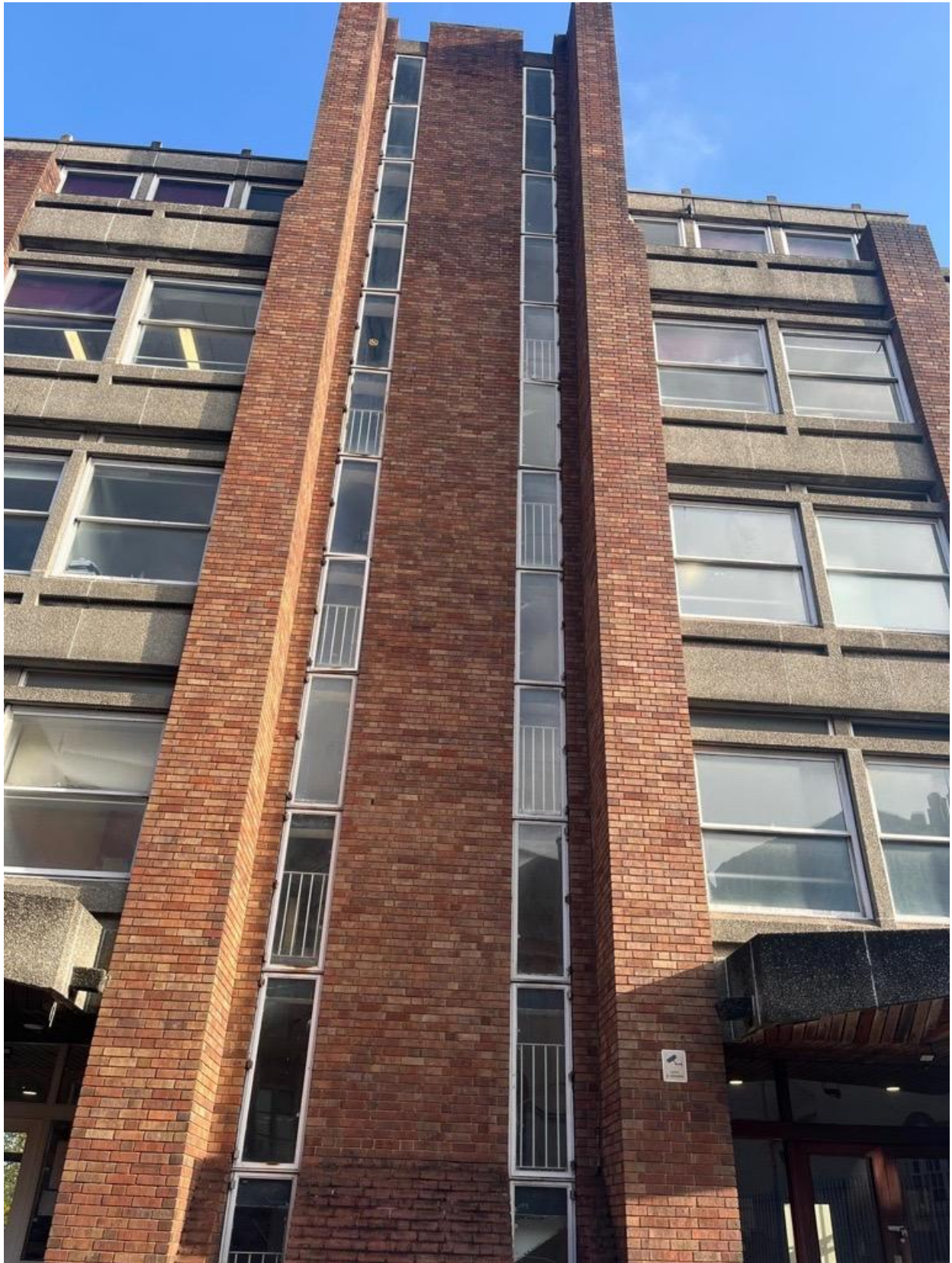
Figure 4 - Window Type 4 (tall rectangular windows on the staircase)
