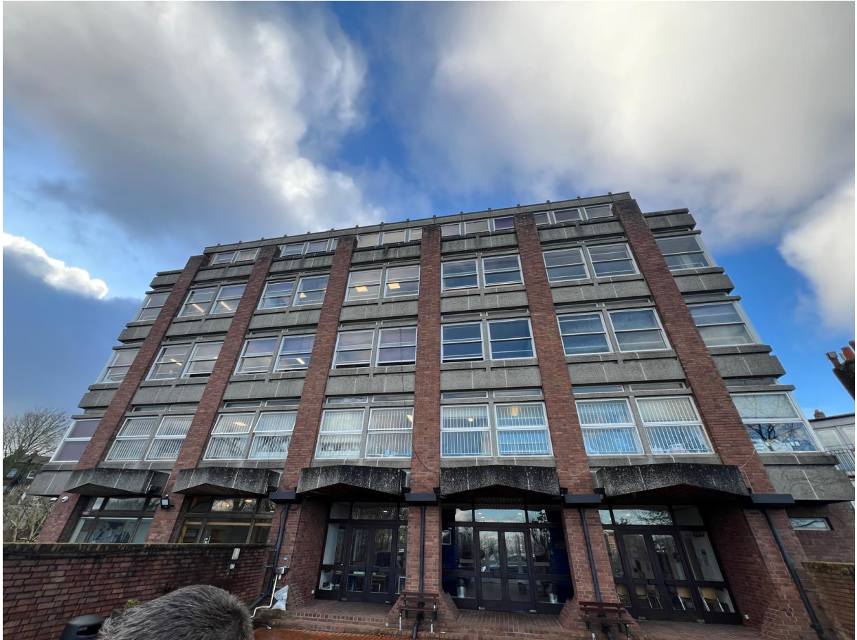
Figure 1 - Rear Elevation comprising of window types 1, 2, 3 and 5
