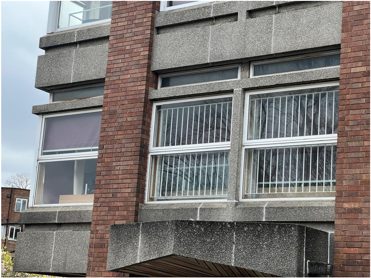
Figure 2 - Close up of window types 1 & 2
