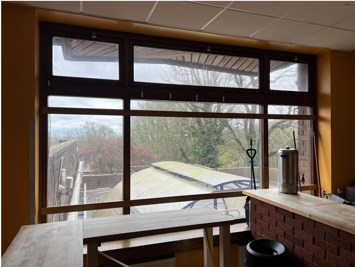
Figure 3 - Internal photograph of the existing window type 3
