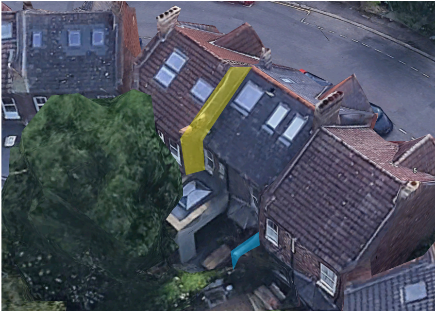
The stepping in the houses means that the rear roof and external wall of 4 Clyde circus is set back from 3 and 5 (highlighted in yellow). The brick wall between 4 and 5 is also shown here (highlighted in blue) and the existing outrigger.
