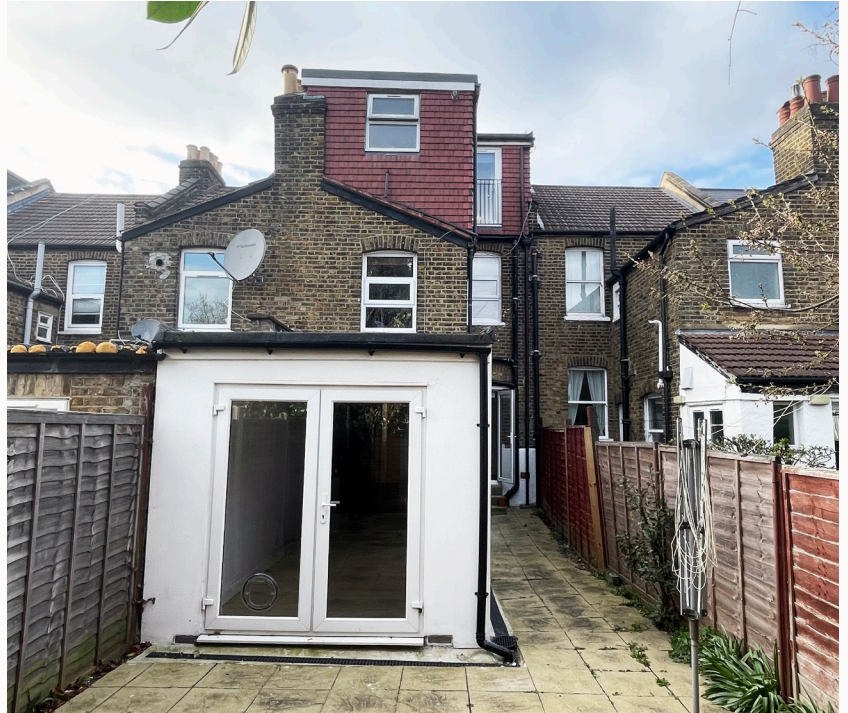
EXISTING REAR FACADE
