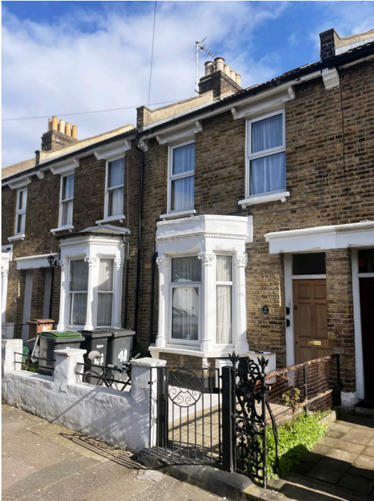
EXISTING FRONT FACADE
