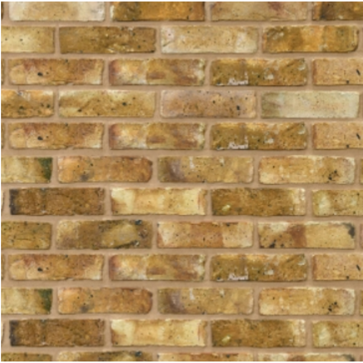
Image – Photo – London stock masonry
