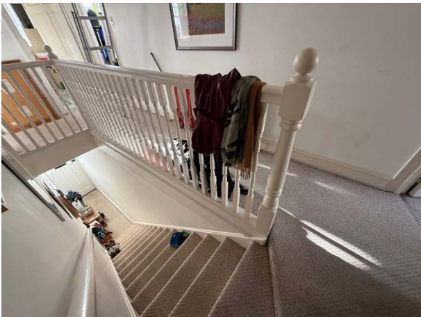
view of the stair access to first floor level
