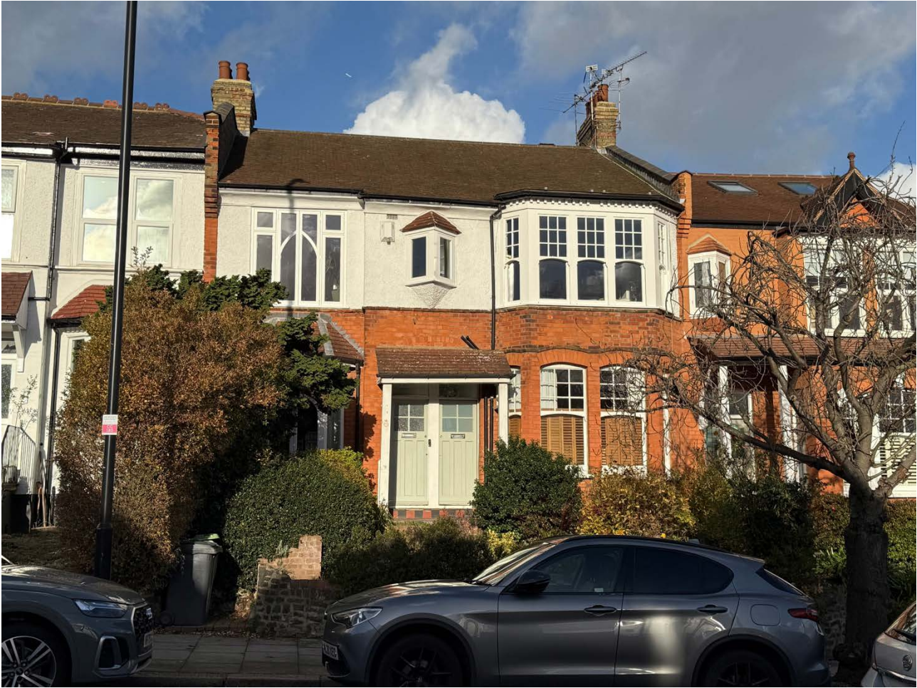
view of the front elevation
