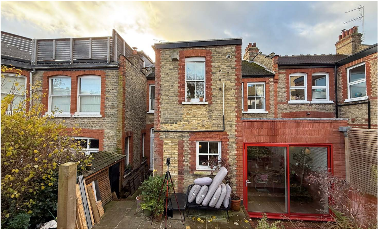
view of the rear elevation
