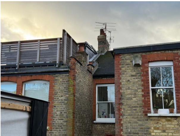
view of the rear elevation parapet wall to No.48
