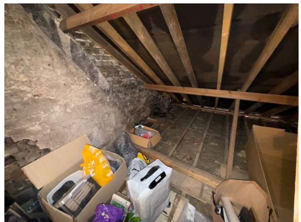
view of the existing loft
