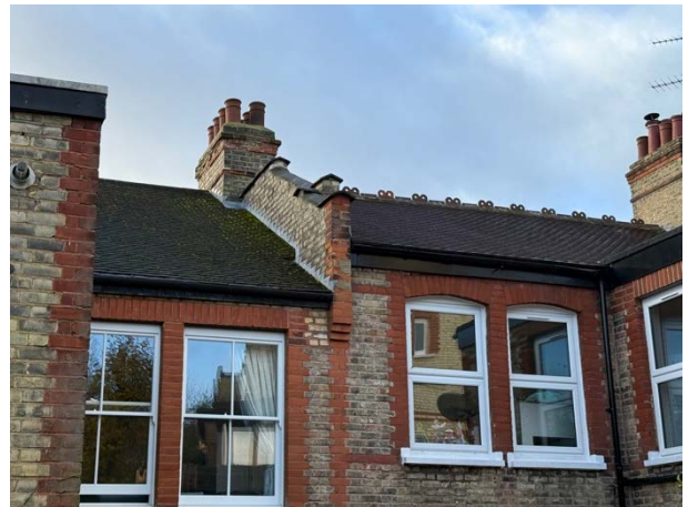
view of the rear elevation parapet wall to No.44
