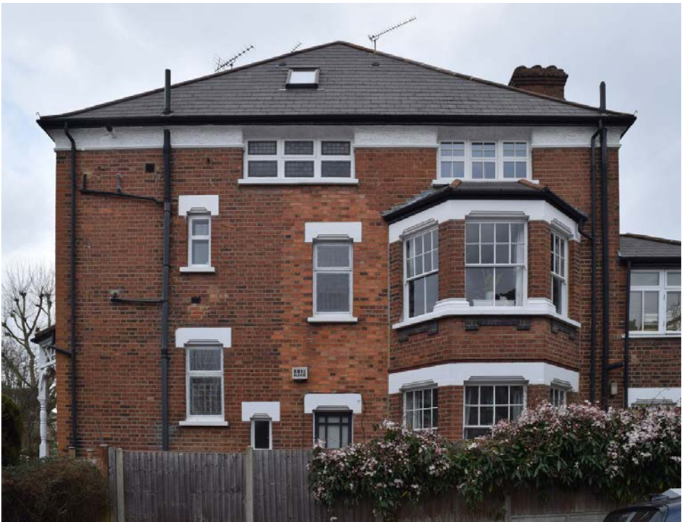
(3) View of 202 Muswell Hill Road from Church Cres (image taken 03/26)
