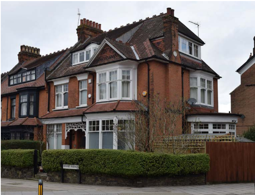
(4) View of 2 Grand Avenue from Muswell Hill Road taken (image taken 03/26)
