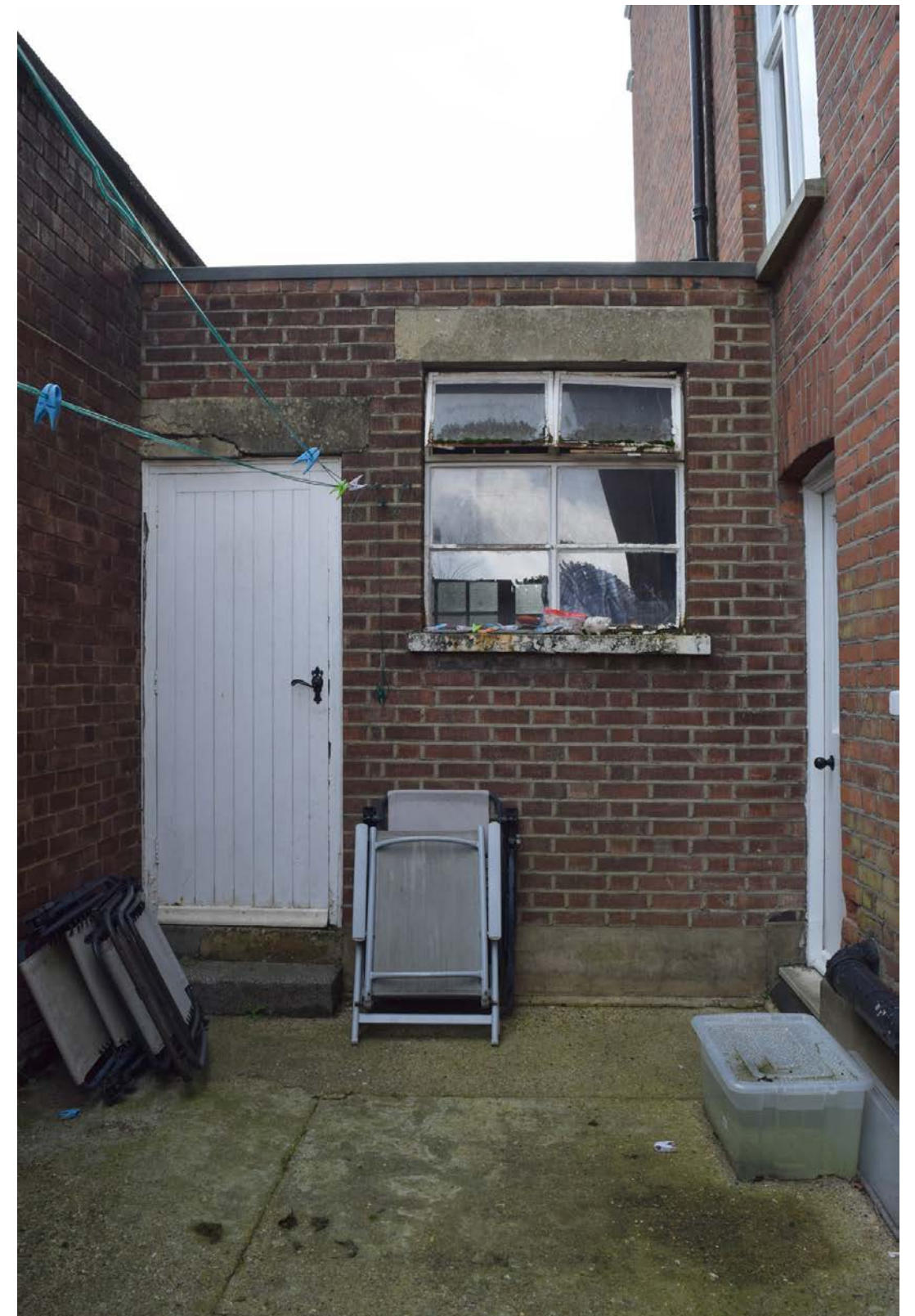
View of the existing garage from the rear garden (image taken 03/26)
