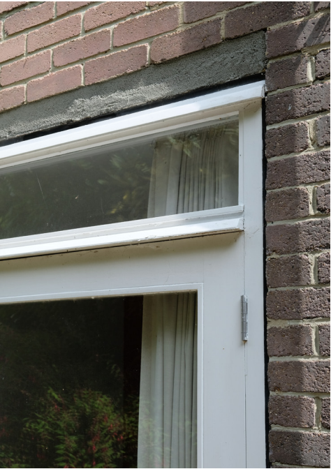
Existing white-painted windows/doors at 25 Hillside Gardens.
