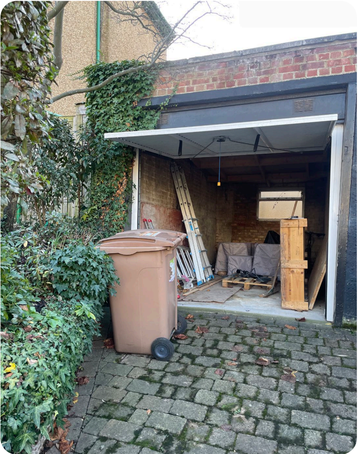
Garage Front Elevation (Close-Up)
