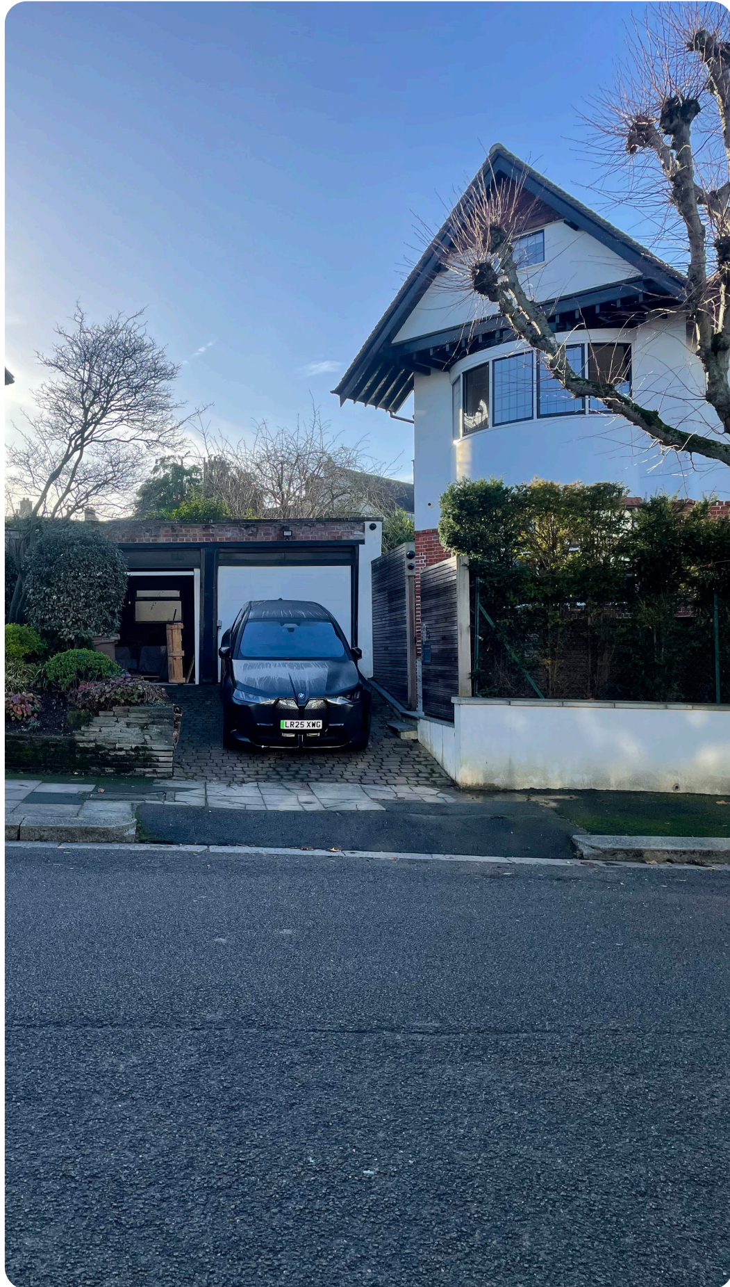
Photographs of the Garage at 55 Vallance Road
