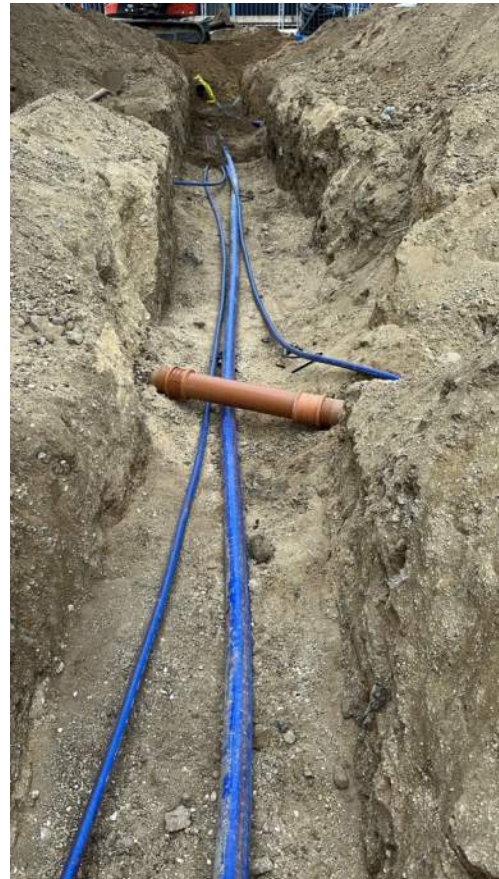
Water Pipe Installation Trench 02
