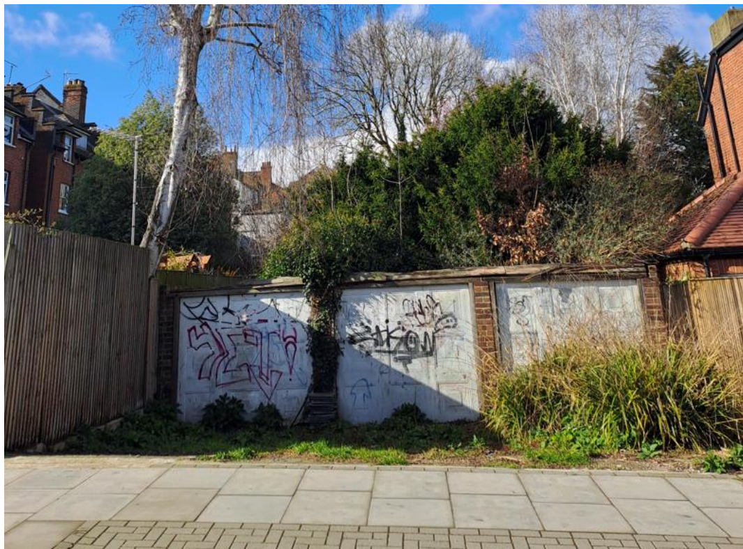
Photo 1 – looking north at the garage. Note the silver birch on the left hand side has consent to be removed.
