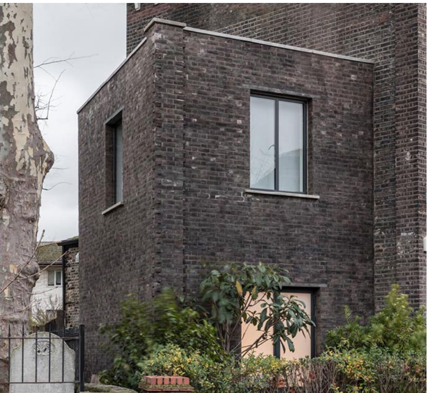
Refined architectural detailing - copings and sills
