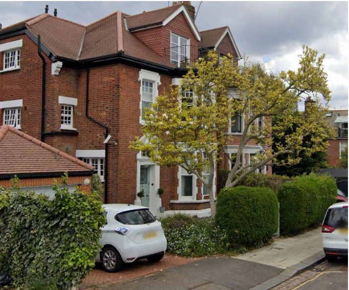
Image of 2 Coleridge Road showing the visibility of the front drive from the street.
