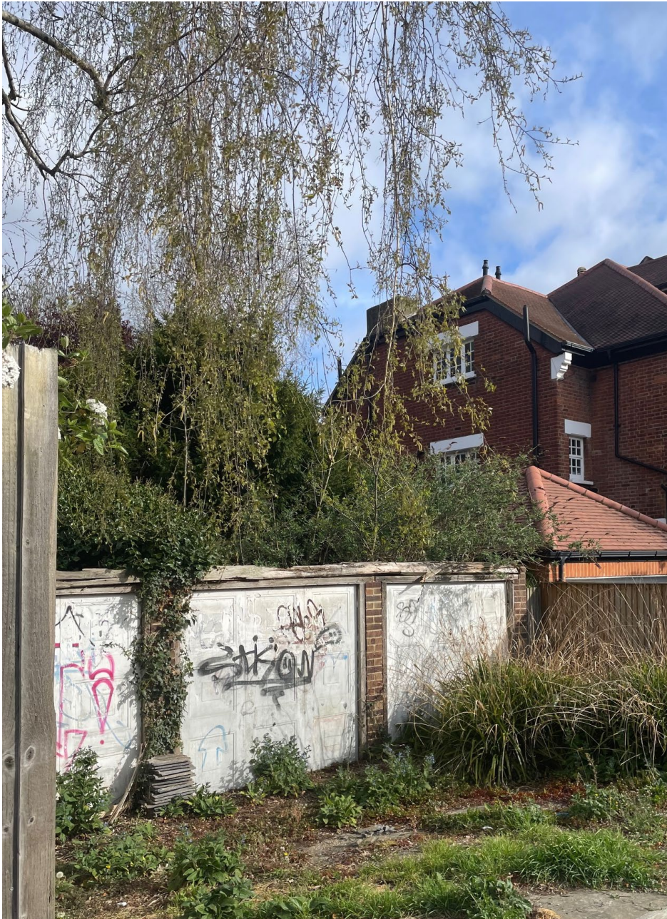
Existing driveway and eastern boundary fence Photographs taken on 25.03.2025
