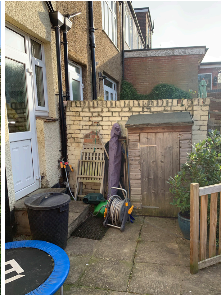
Looking towards the neighbouring properties from the porch. Several properties feature rear extensions.
