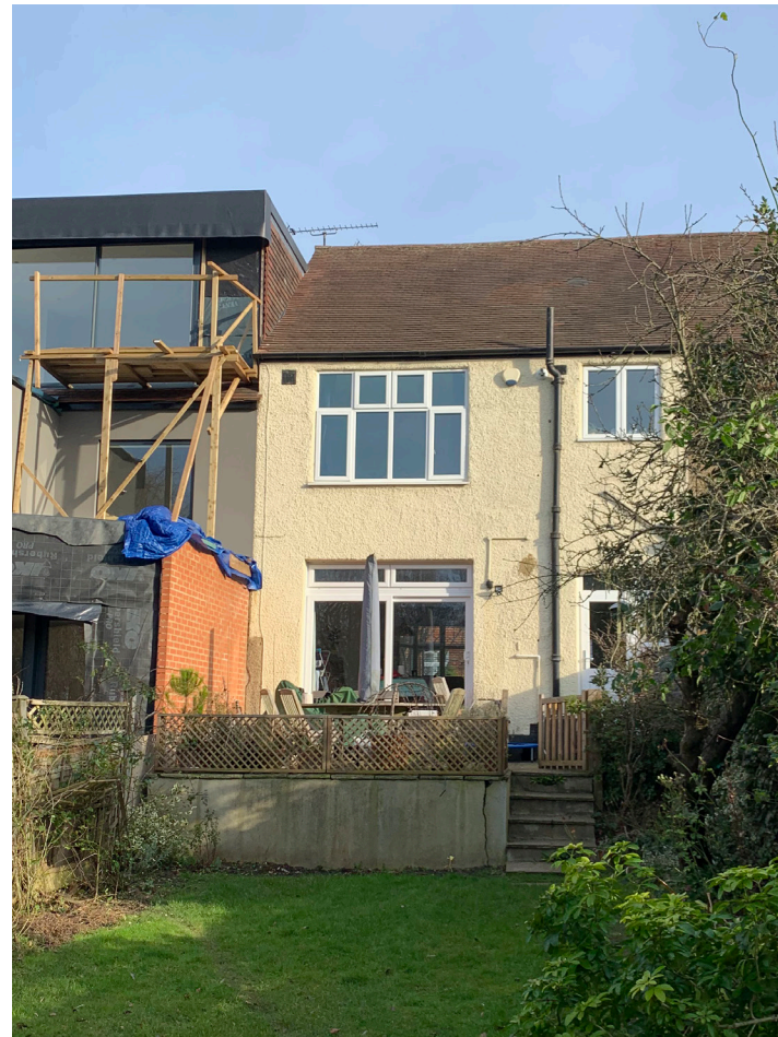
Rear of the house. Several steps lead up to the raised patio. The extension at 159 Higham Road is currently under construction (HGY/2019/1004).
